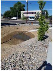
3. The pond also needs to be reshaped at the outfall sidewalk culvert per the approved plans. Currently the pond cannot discharge into the sidewalk culvert.
