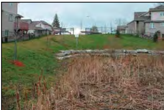
Fully Established, Functioning Rain garden
