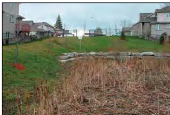
Fully Established, Functioning Rain garden
