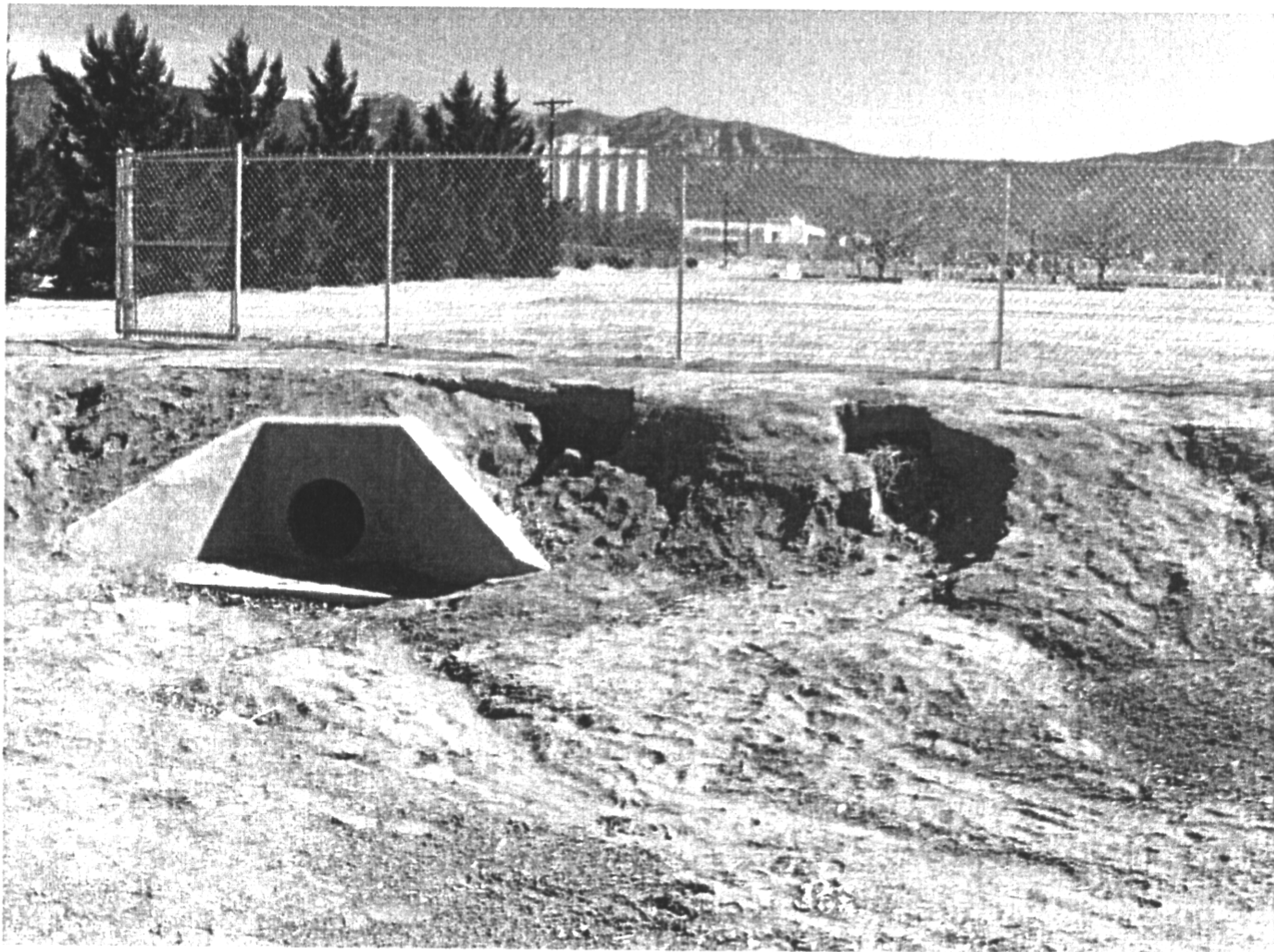
Photo 2 – 24" Storm Drain Outfall to Pond
