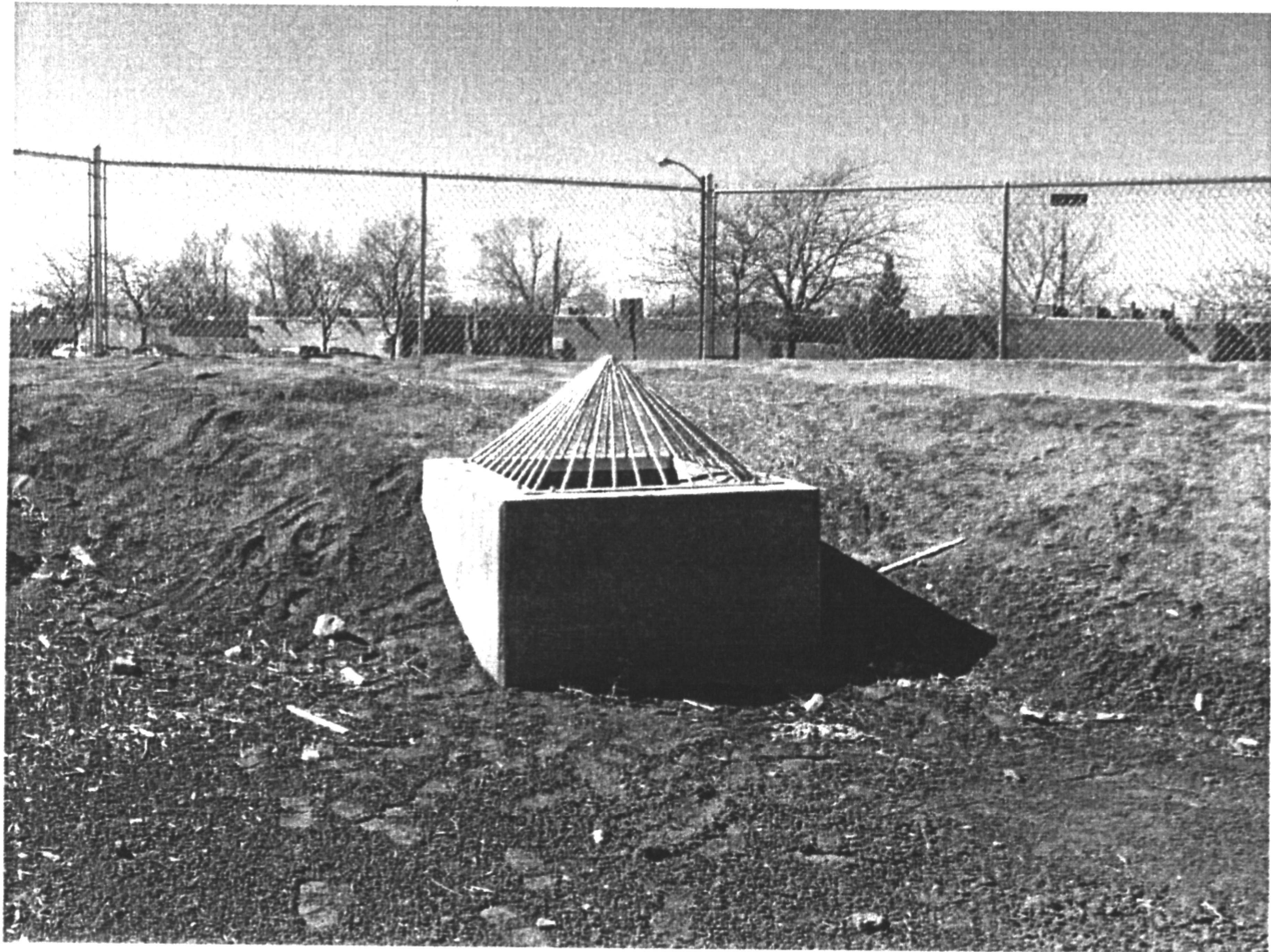
Photo 1 – Retention/Detention Pond Outlet Structure
