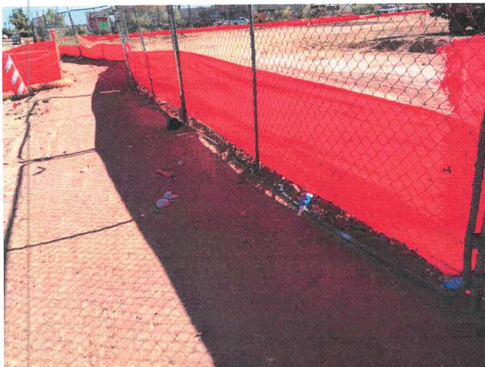
Bury Silt fencing 6" below grade
