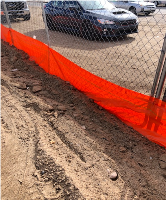
Silt Fence Established Along Perimeter
