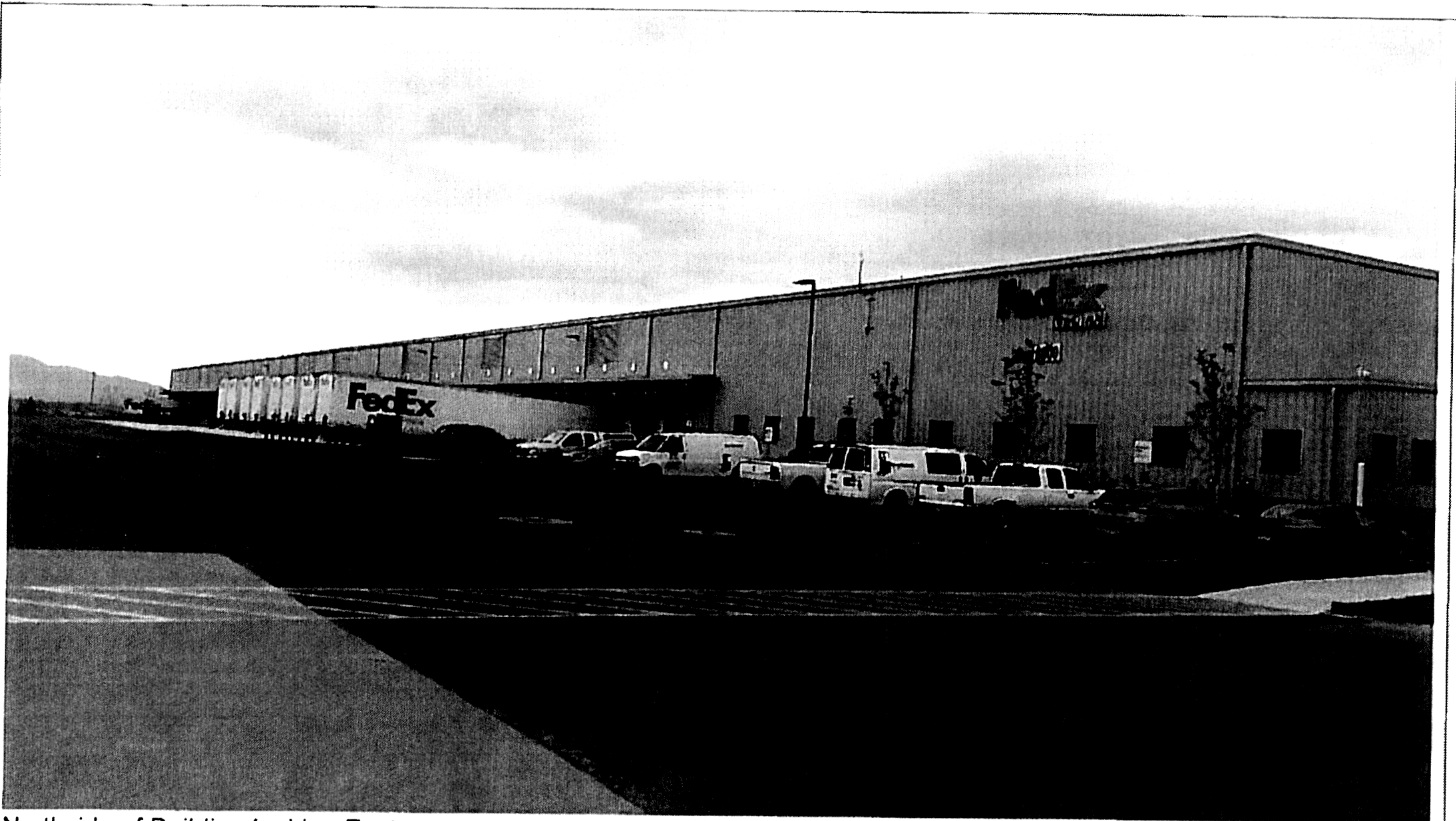
Northside of Building looking East
