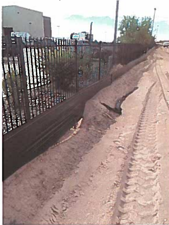
Site Walk Deficiency Photos - East Perimeter: Silt Fence
