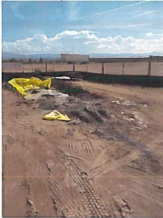
Site Walk Deficiency Photos - concrete washout area
