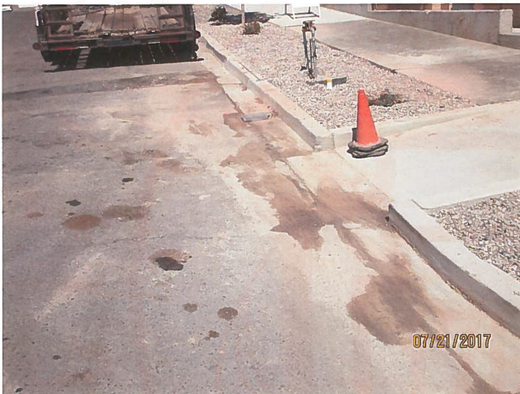
Sediment and oil/hydraulic fluid in area that drains to unprotected inlet.
