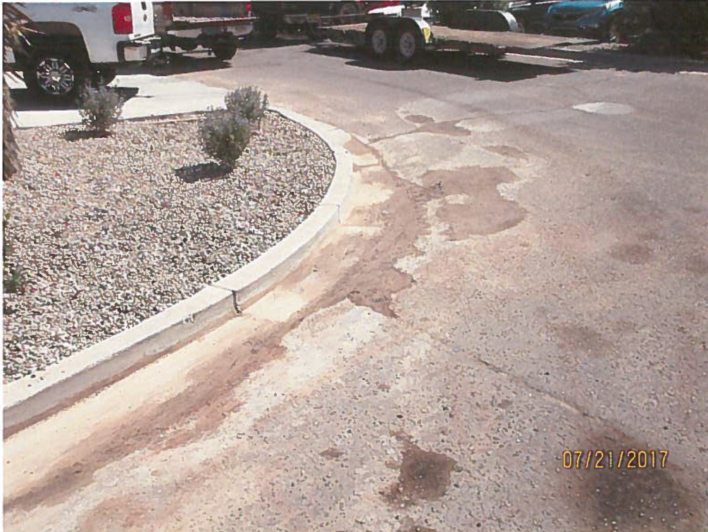
Sediment in area that drains to unprotected inlet.
