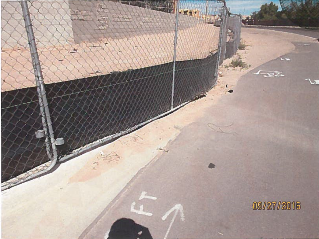
Silt fence not buried at intersection and sediment in street.
