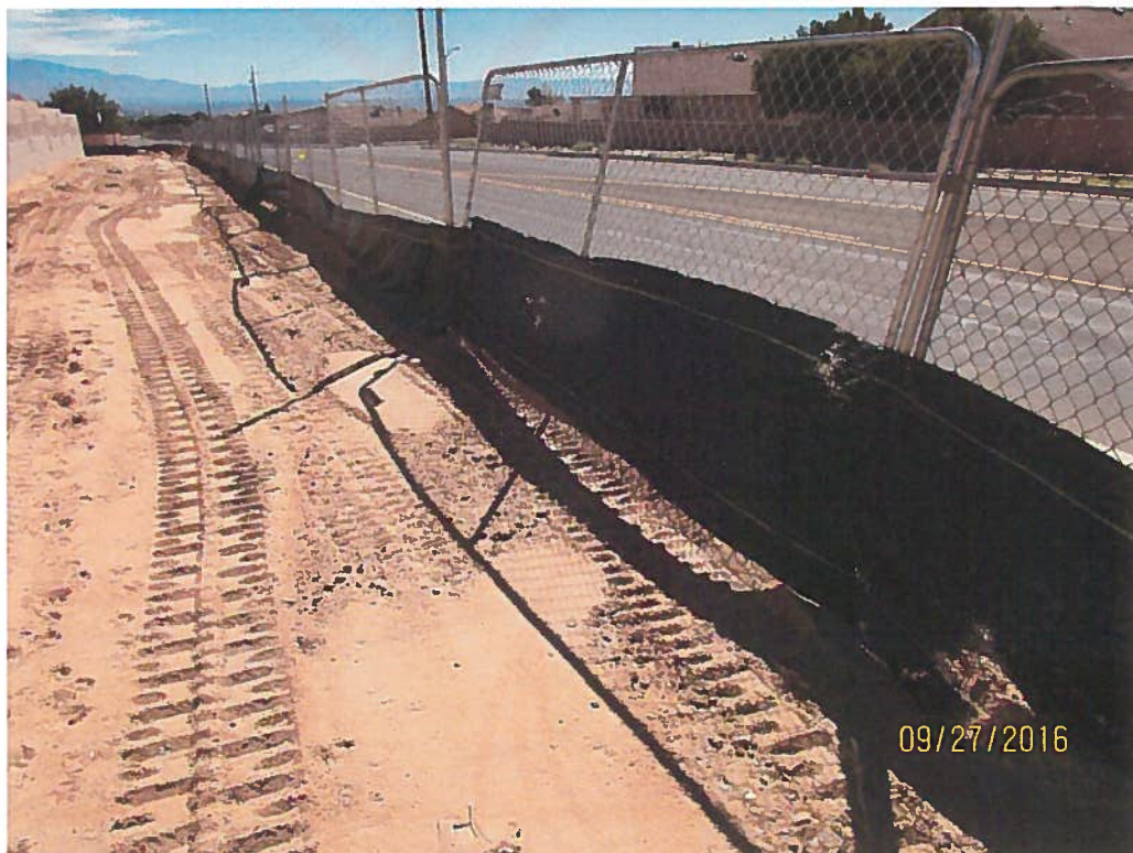
Silt fence not buried on Bluewater Rd.
