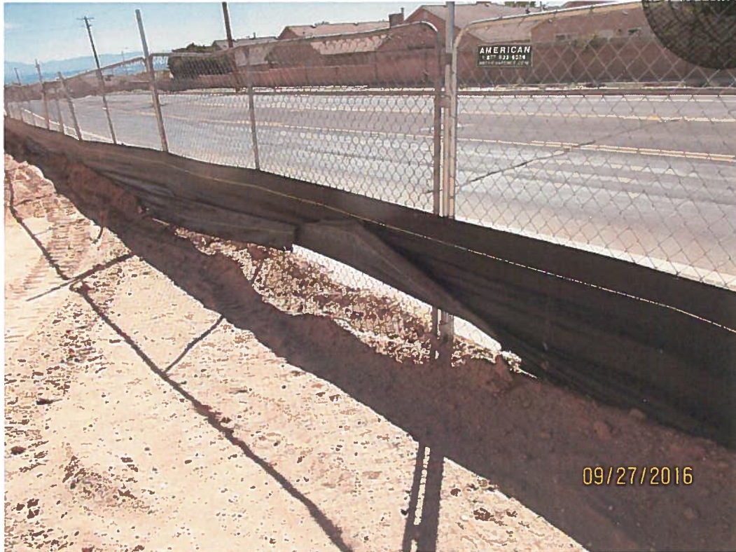
Silt fence tied-up above the ground on Bluewater Rd.
