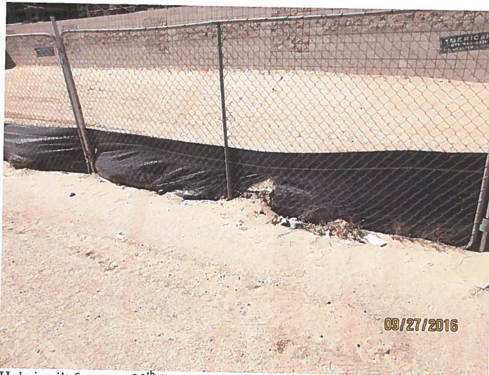
Hole in silt fence on 90 th St.
