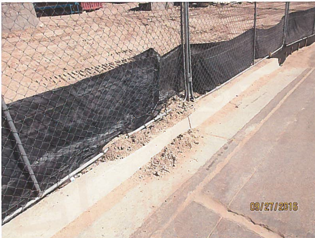
Silt fence not buried and sediment in Bluewater Rd.
