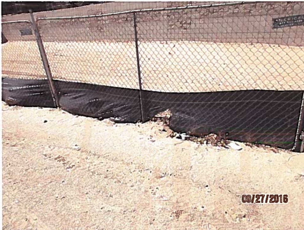
Hole in silt fence on 90 th St.
