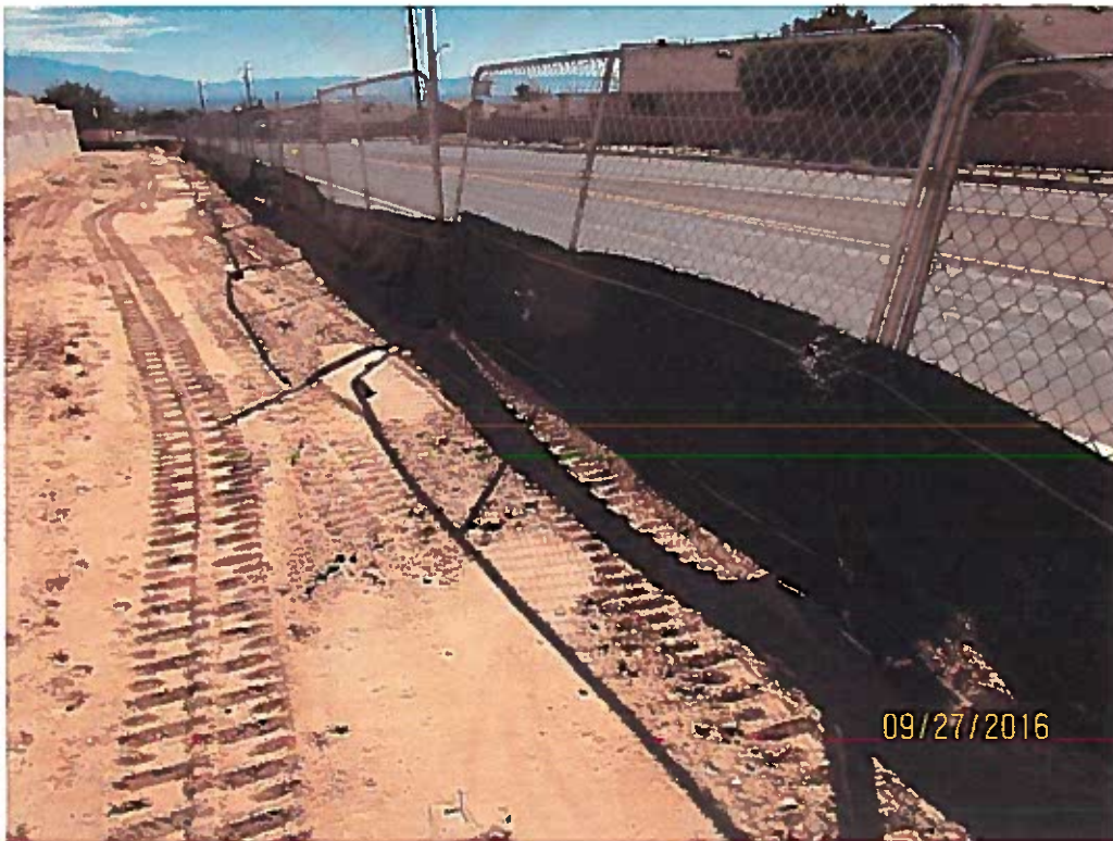
Silt fence not buried on Bluewater Rd.
