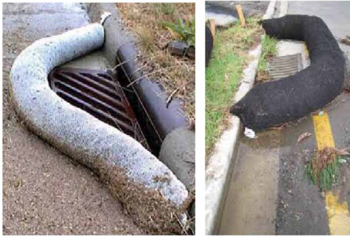
Curb Storm Inlet Protection with Wattles
