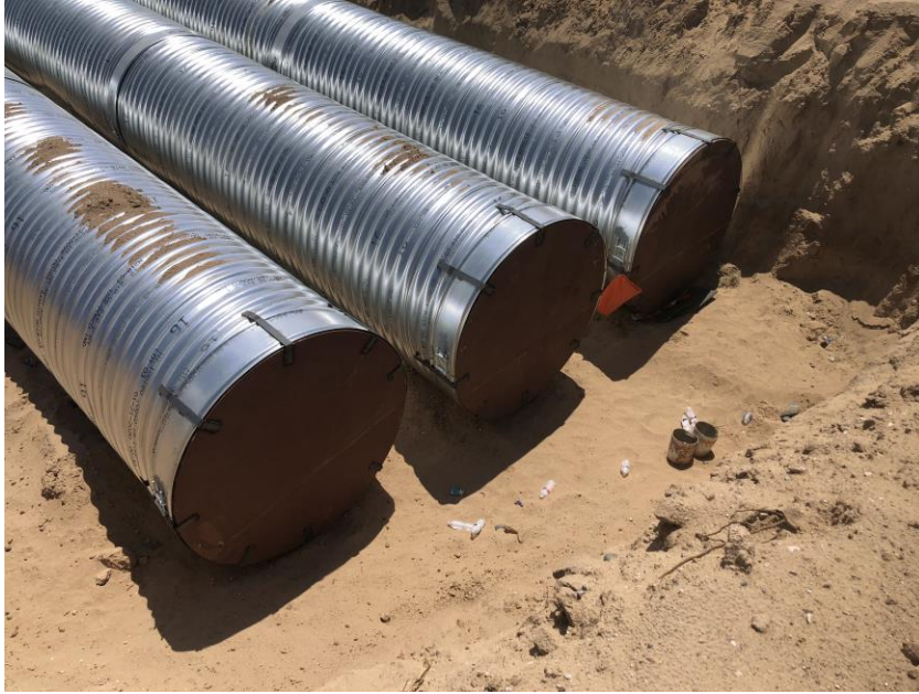
Installation of 72" culverts – east end
