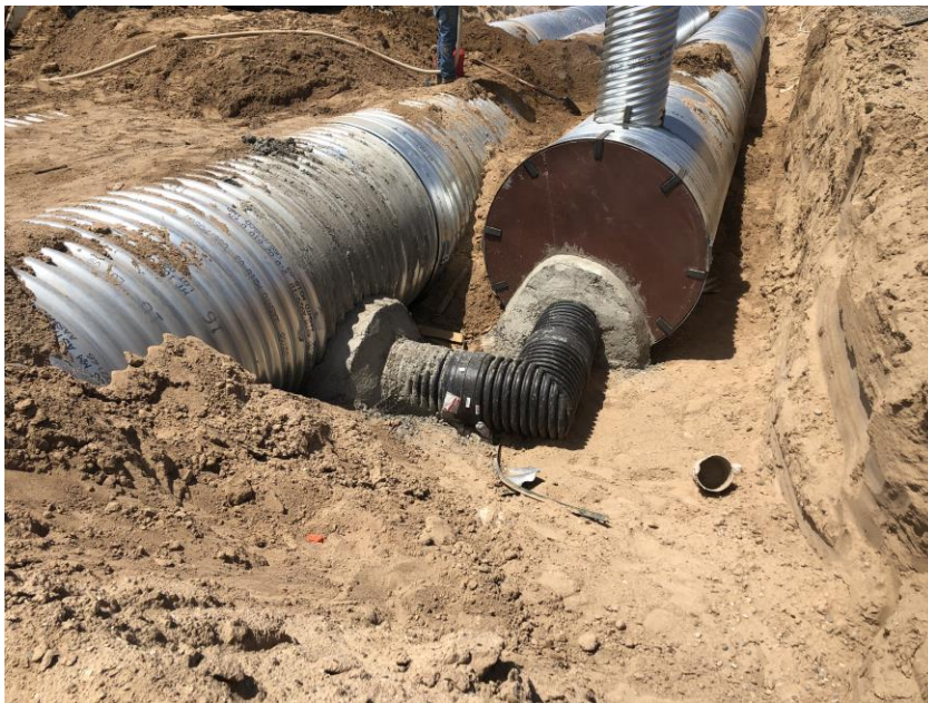
Water quality MH and 72" culverts with bulkheads
