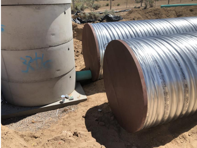
Connector pipe between 72" culverts at mid-run
