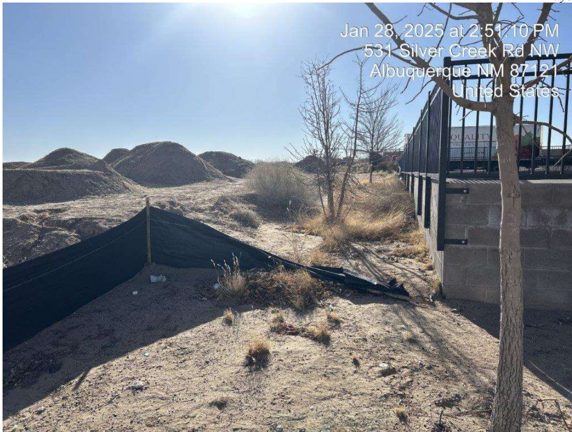
4 Collapsed silt fence
