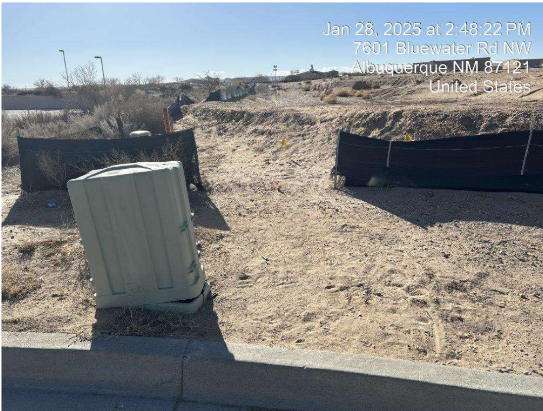
2 Missing section of silt fence from 1/28/25
