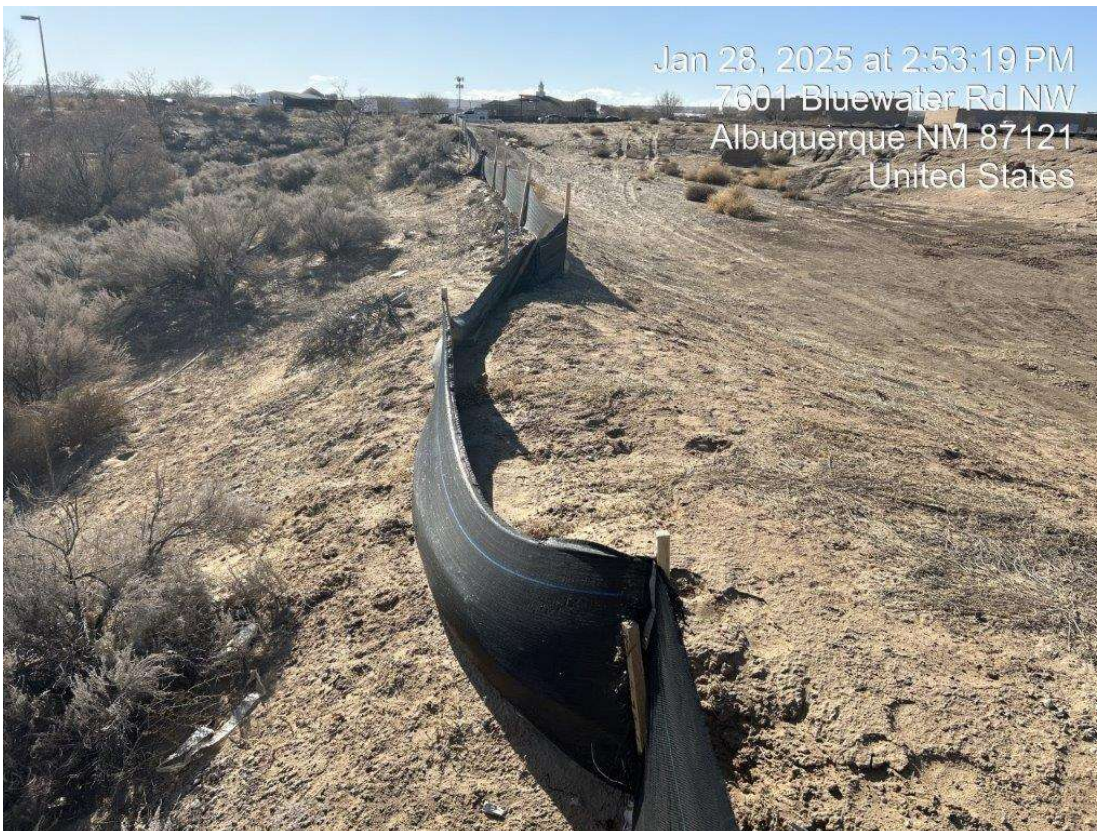
3 Silt fence over one-half of the above-ground height
