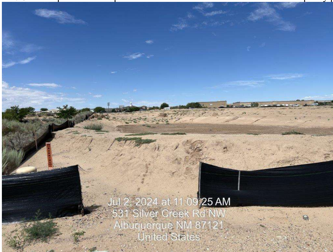
1 Missing section of silt fence from 7/2/24
