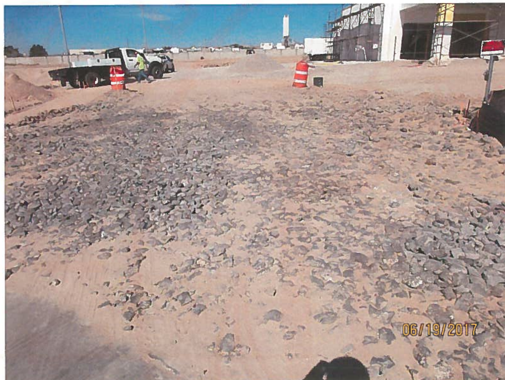
Track-out pad requires maintenance.
