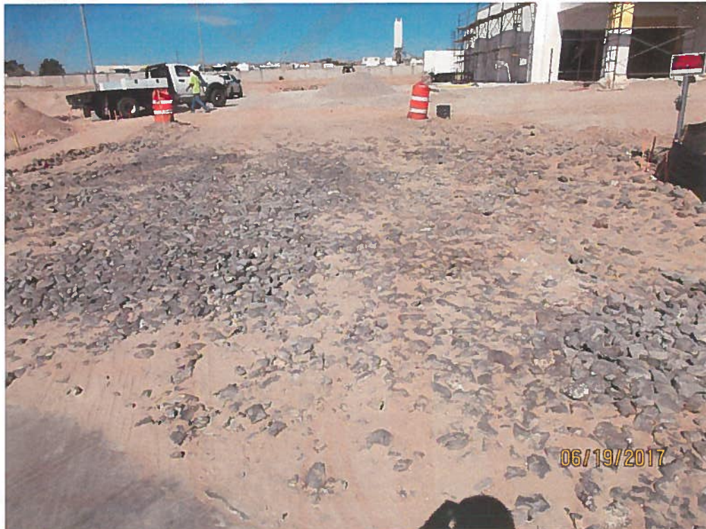
Track-out pad requires maintenance.
