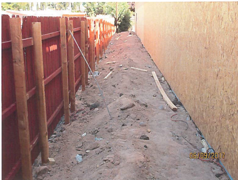
Dirt pile west of building. No sediment BMP.
