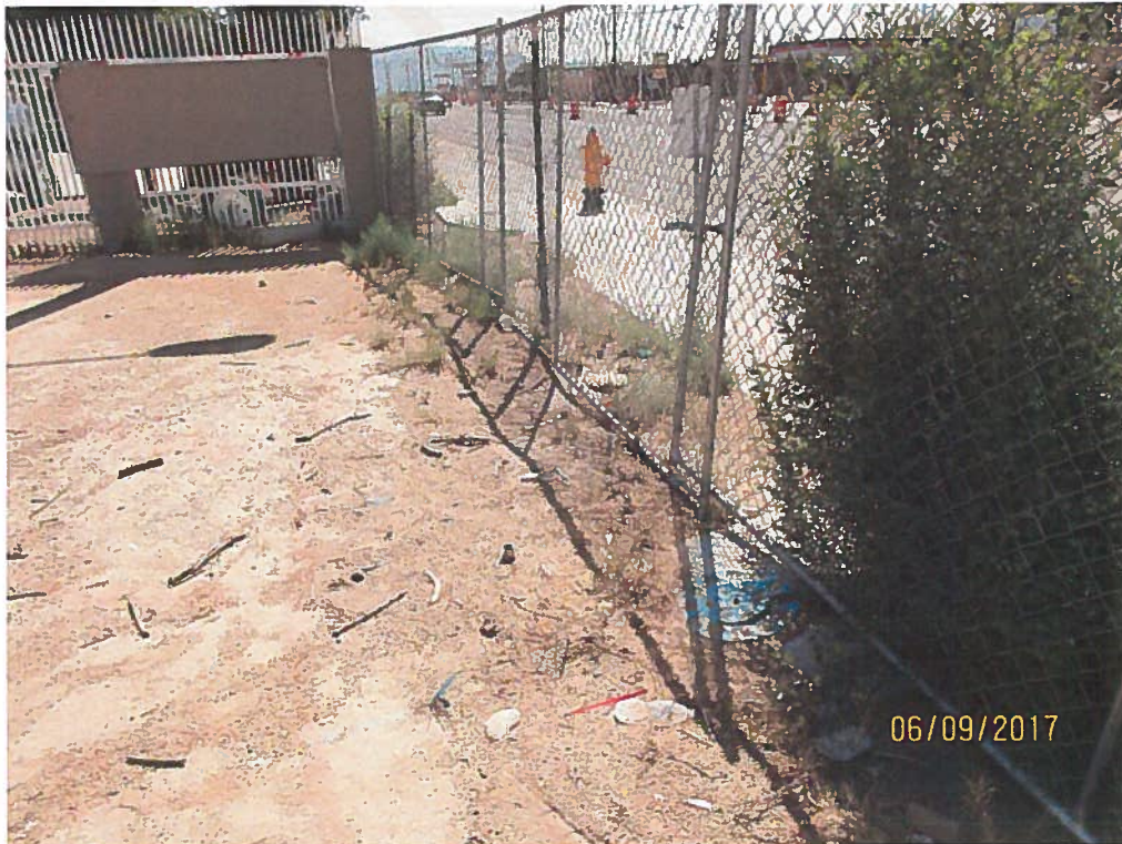
No silt fence and trash.
