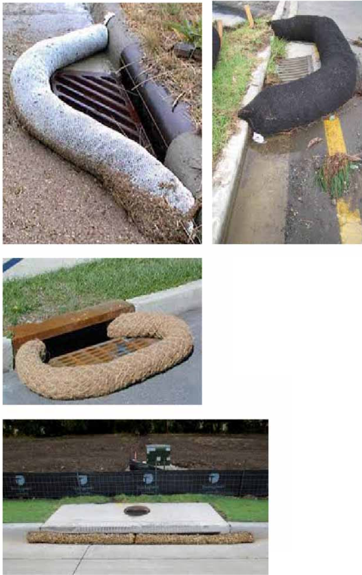
Curb Storm Inlet Protection with Wattles
