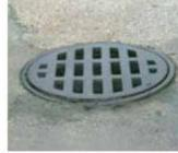
1. Remove sediment, debris, ice and snow from the inlet grate surface and surrounding area.
