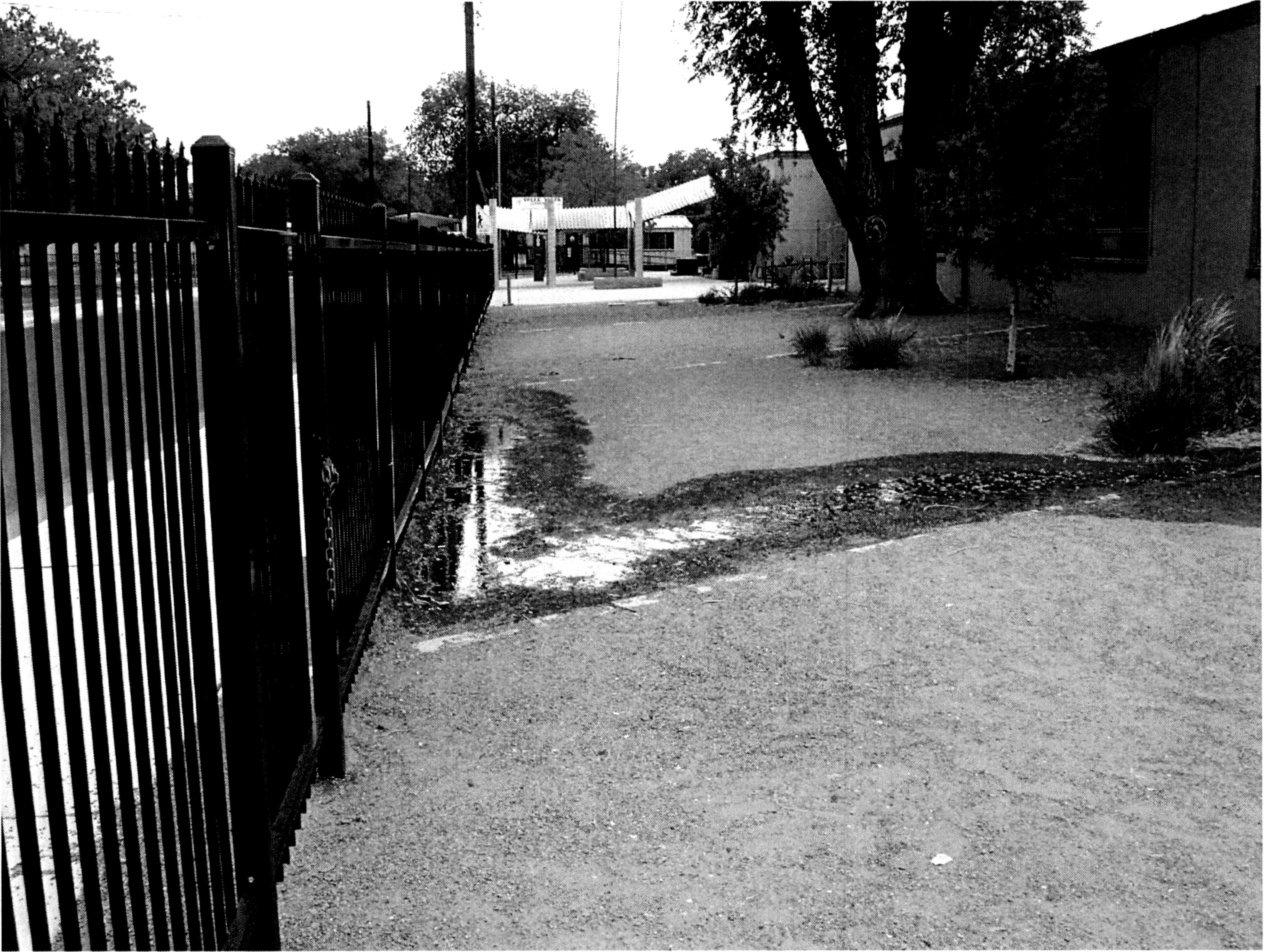
FIGURE 4: Close-up view of existing drainage problem that can be solved by minor re-grading and sidewalk culverts. Date of photograph 05-01-2011.
