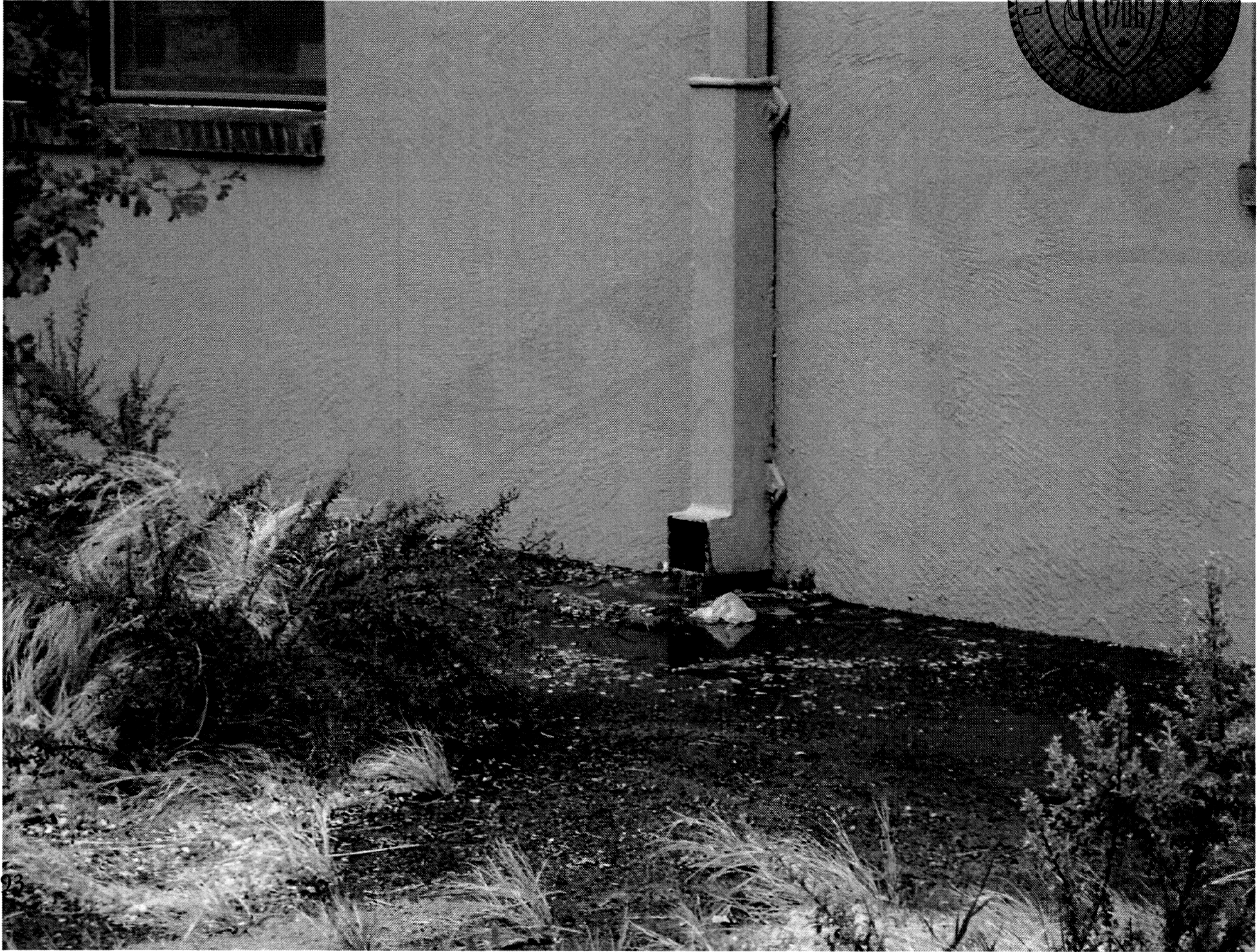
FIGURE 5: One of 3 existing roof drains that discharge to the landscaped area. Date of photograph 05-01-2011.
