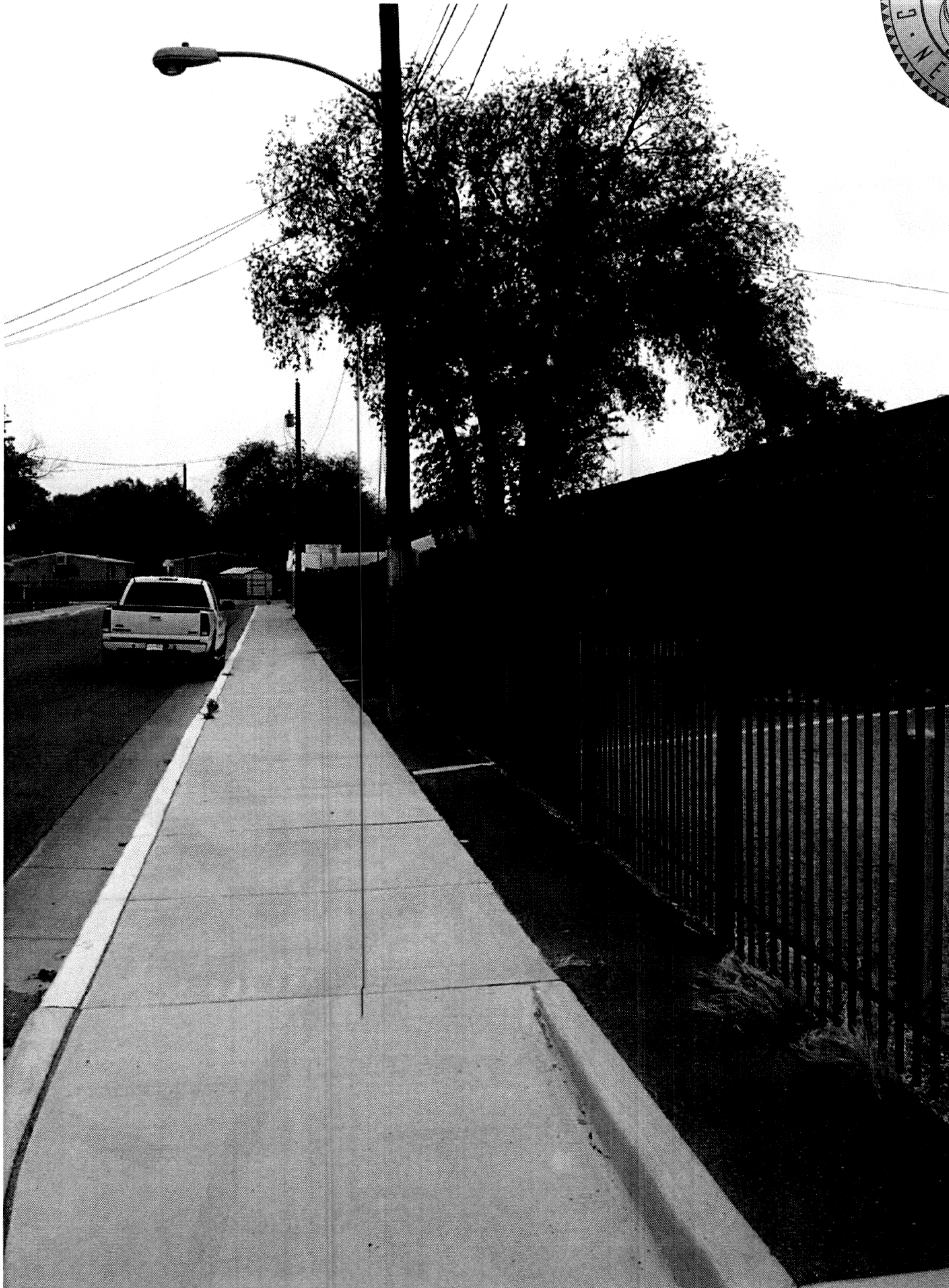
FIGURE 1: South curb line of Mae Street SW with 6' City sidewalk at back of curb and asphalt paving from back of sidewalk to fence line. Date of photography 05-01-2011.
