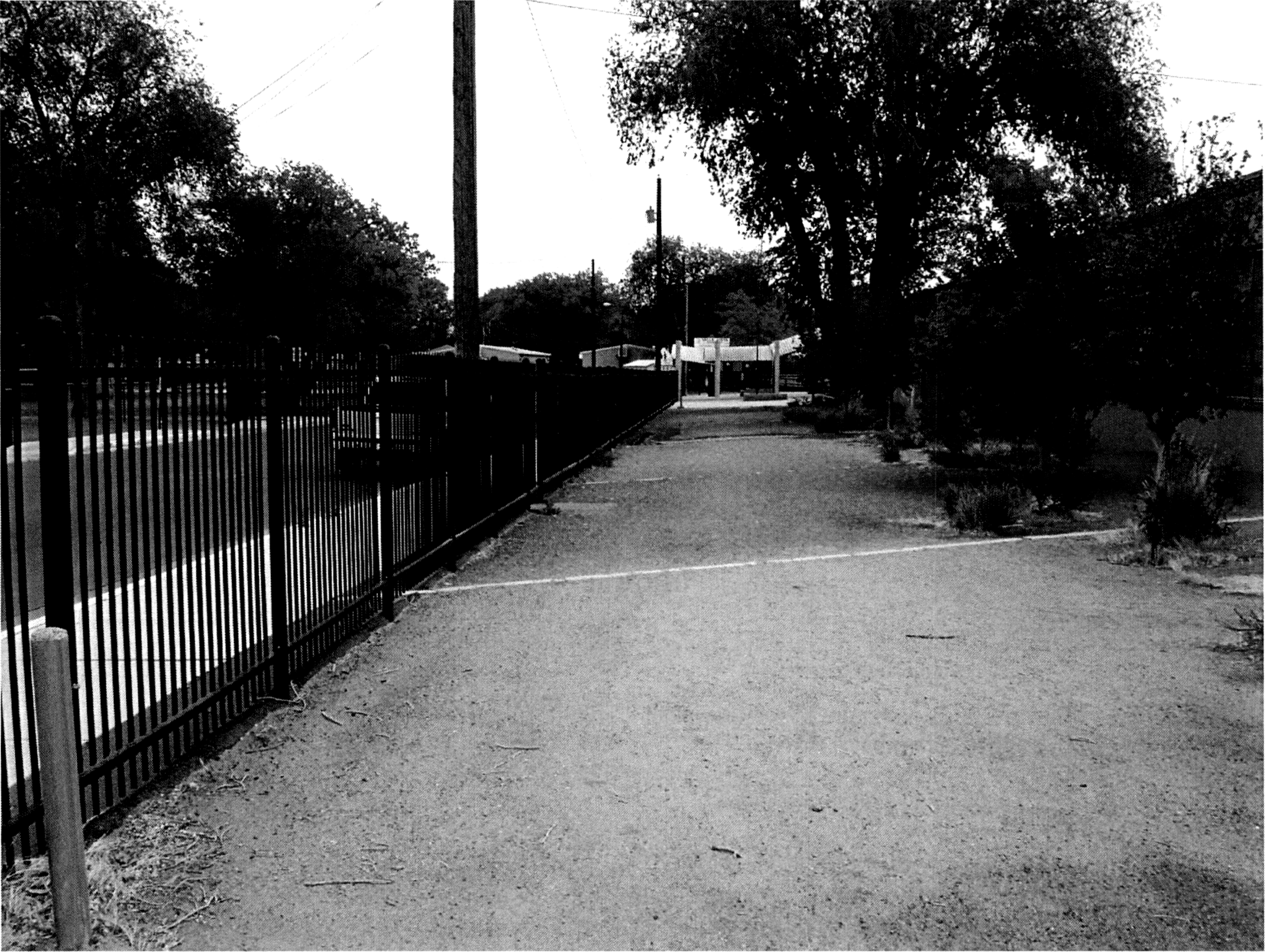
FIGURE 2: View of area behind fence where it appears students wait for the bus. The ornamental fence has 4 existing gate openings and a small asphalt paved pad at each opening. Steel bollards exist at each end; purpose not known. More fencing might be appropriate to control the flow of students across existing landscaping. Date of photography 05-01-2011.
