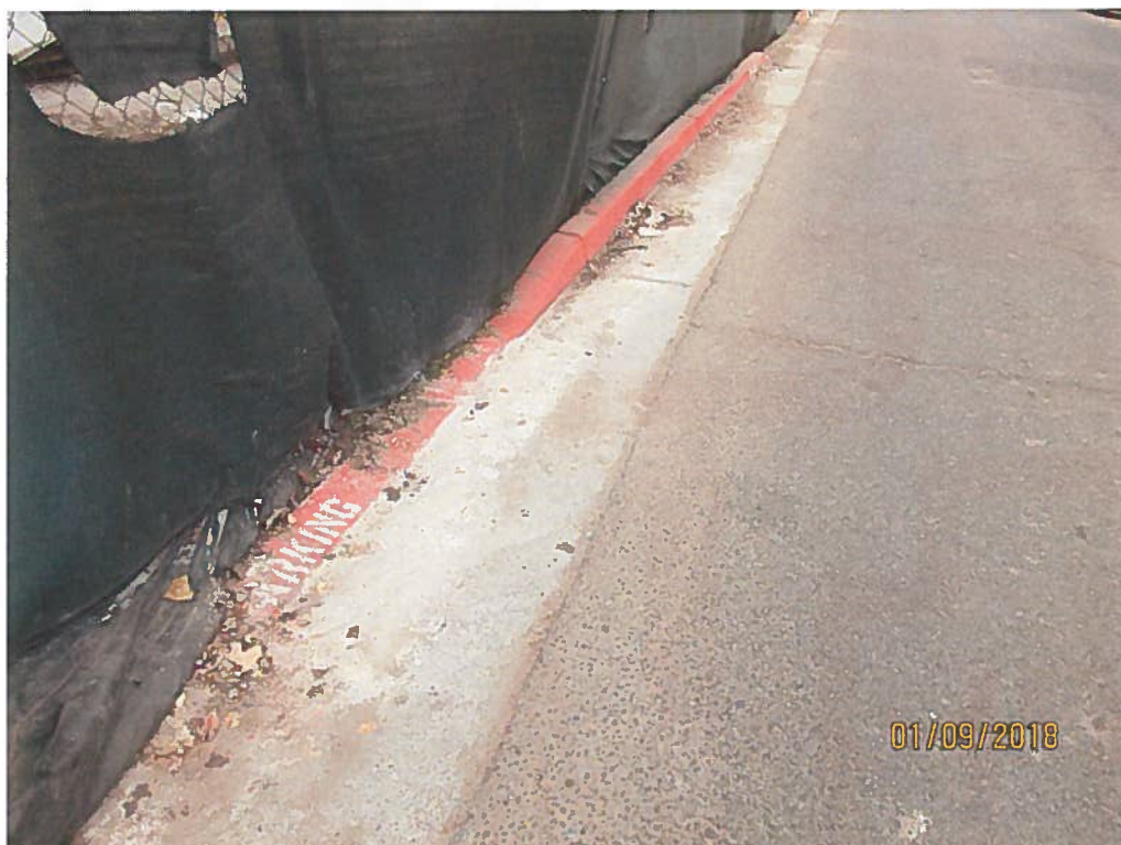
Remnants of wash-out in gutter of Silver Ave.
