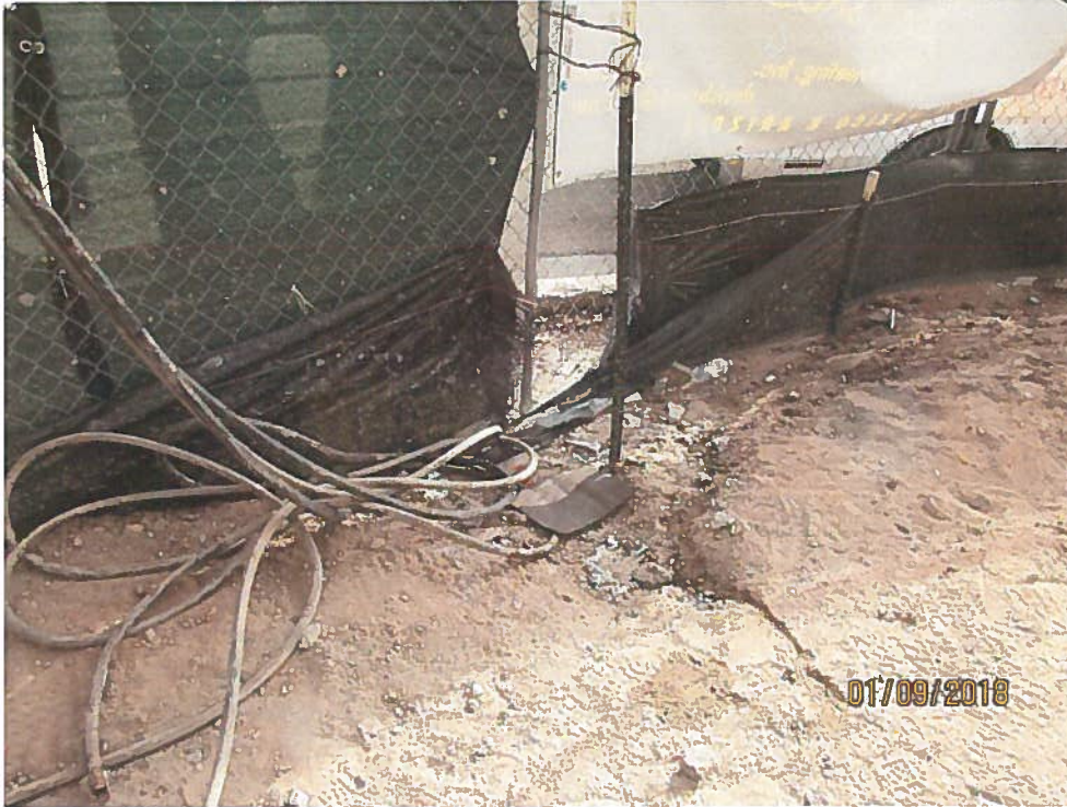
Silt fence requires maintenance.
