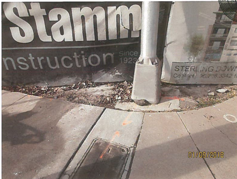
Wash-out draining over sidewalk.
