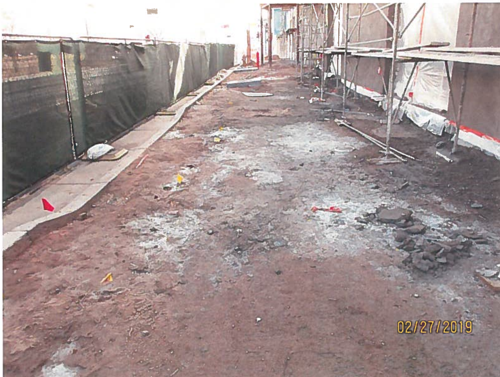
Stucco wash-out on north side of building.
