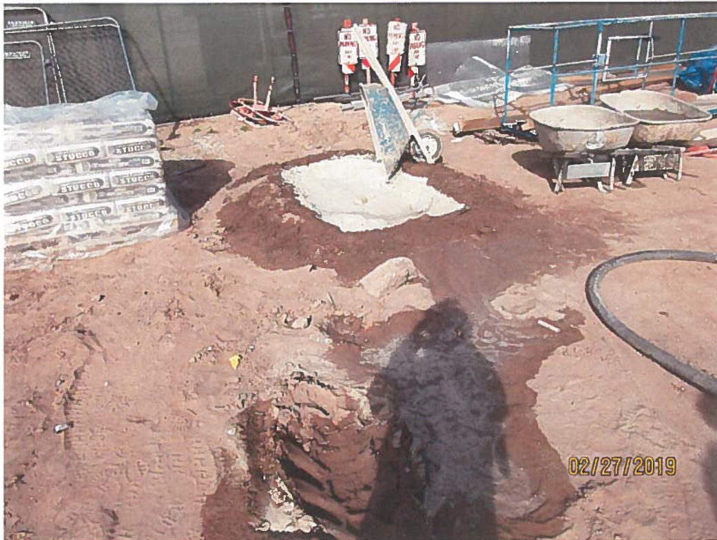
Stucco wash-out in unlined pit.
