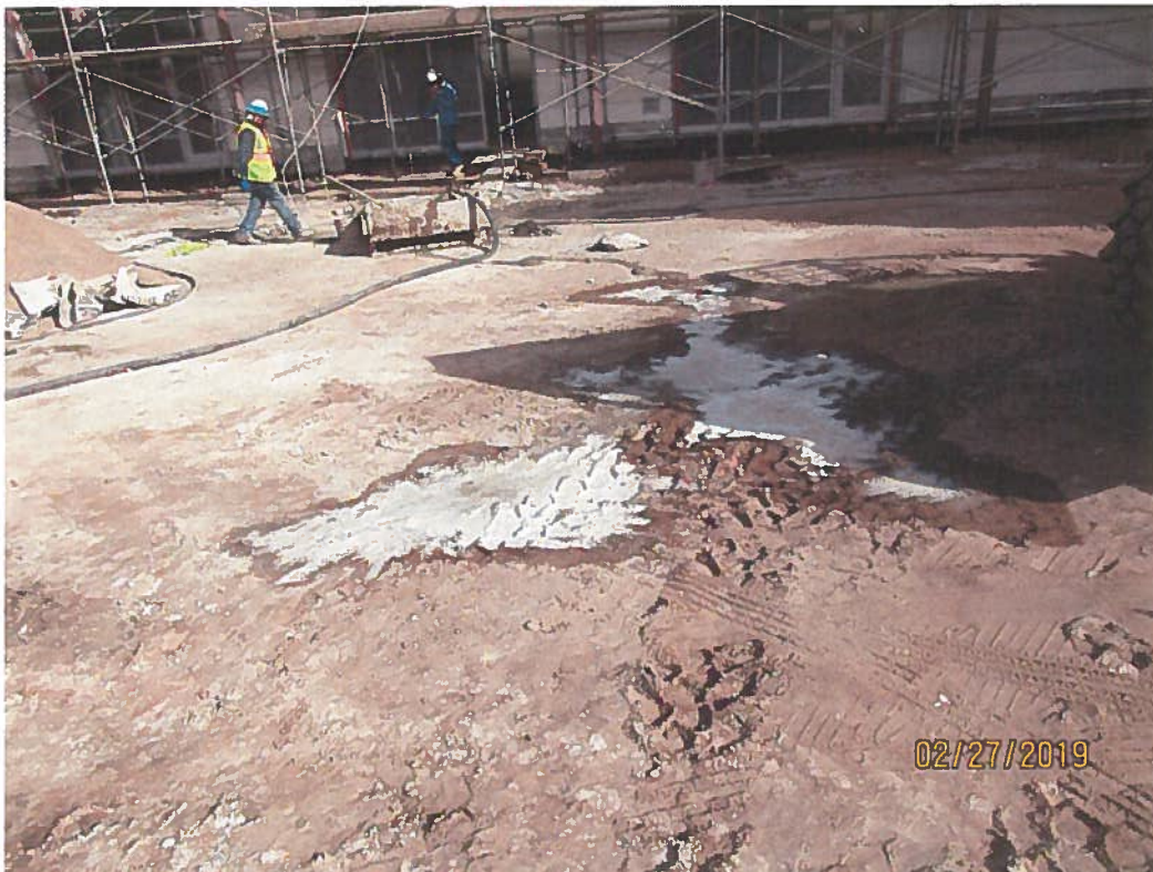
Stucco wash-out on the ground.
