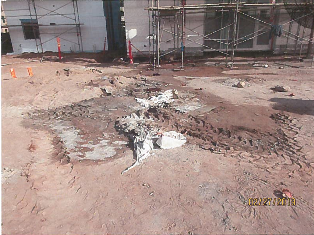
Stucco wash-out on the ground.
