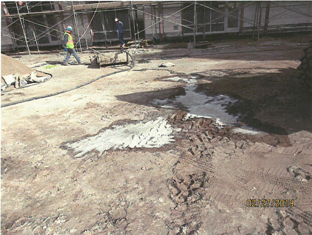
Stucco wash-out on the ground.
