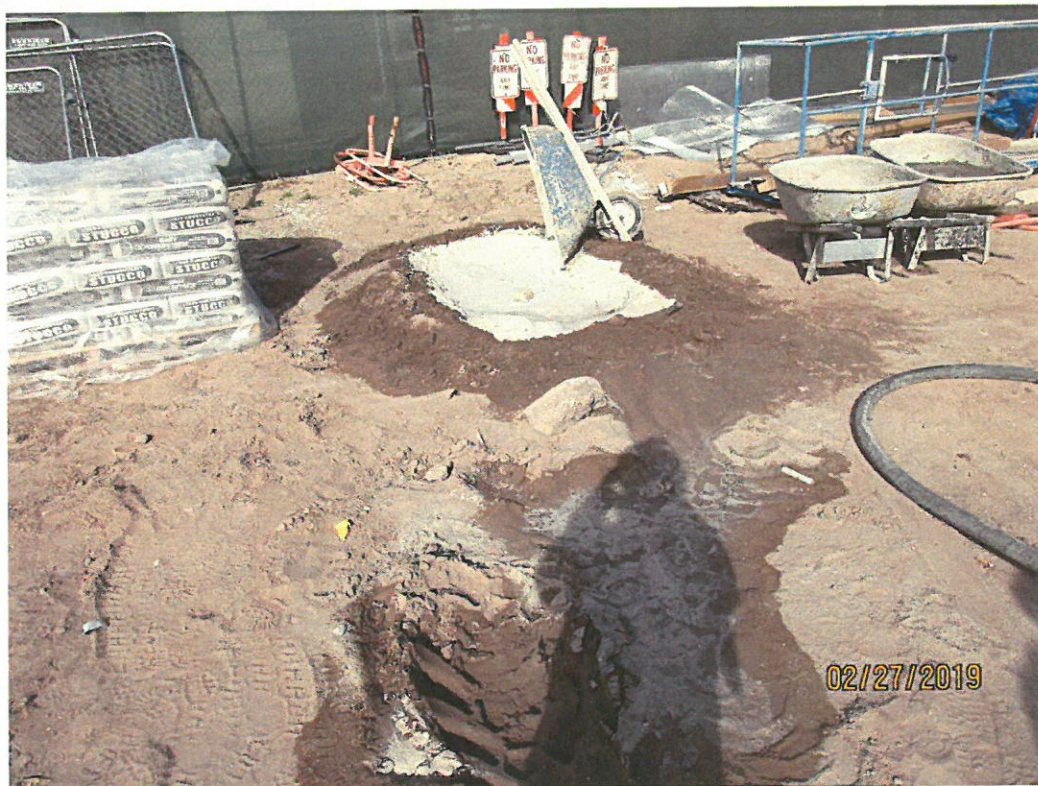
Stucco wash-out in unlined pit.
