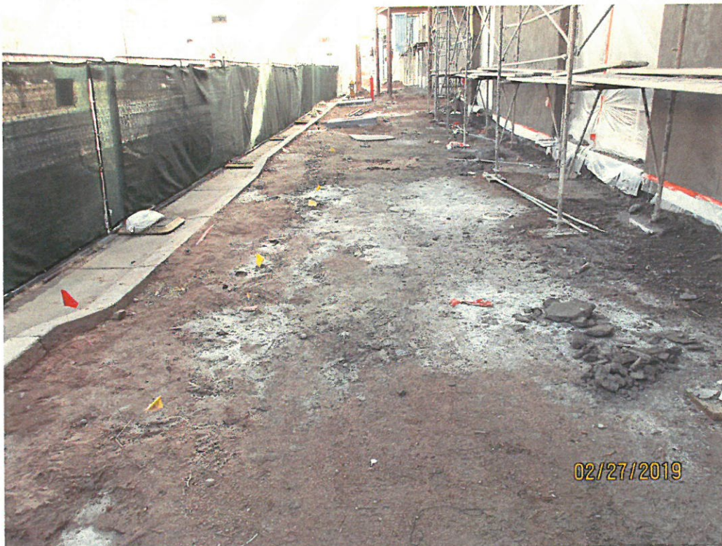
Stucco wash-out on north side of building.
