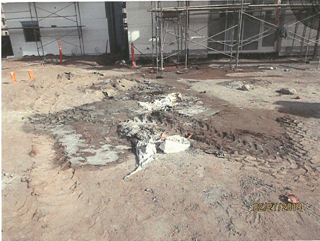
Stucco wash-out on the ground.
