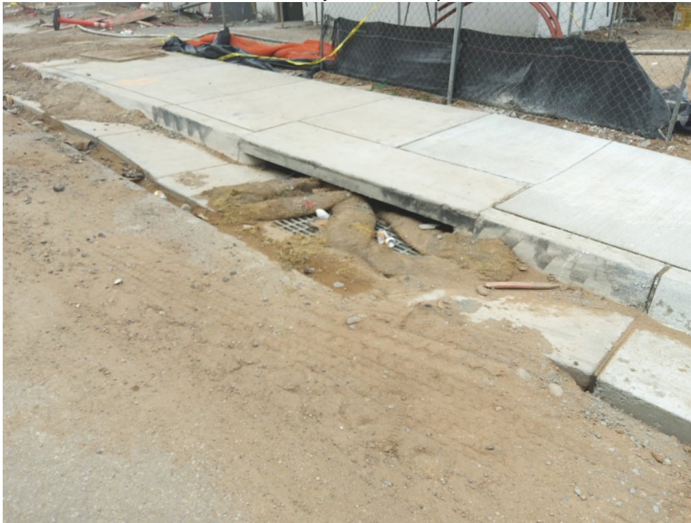
Site Walk Deficiency Photos - Inlet protection
