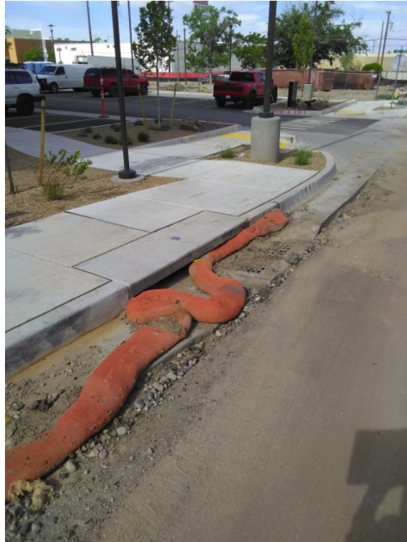
Site Walk Deficiency Photos - Inlet Protection - Mulberry and copper
