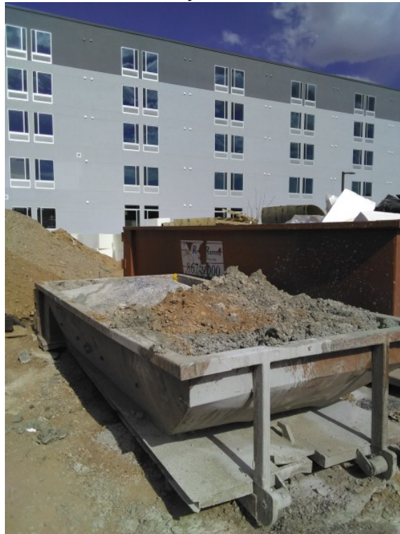
Site Walk Deficiency Photos - Washout Bin
