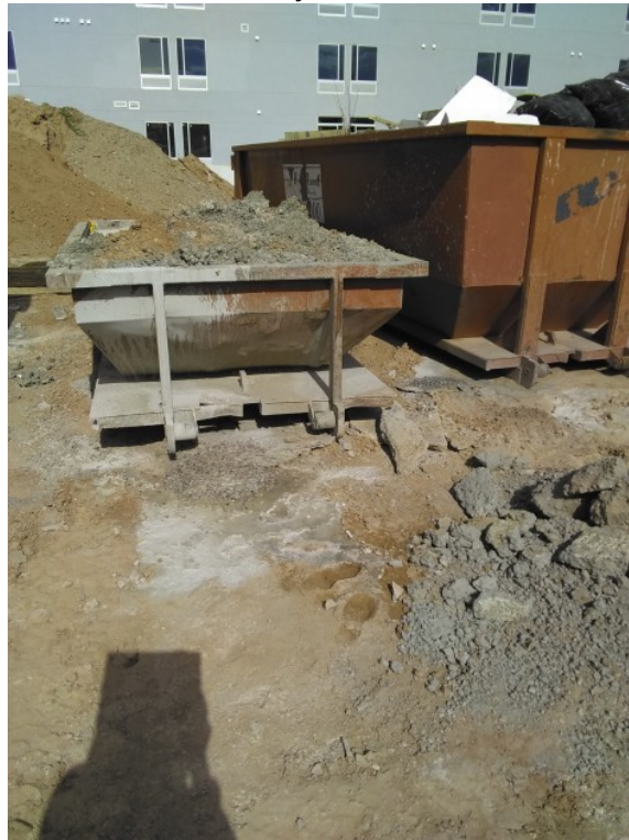
Site Walk Deficiency Photos - Washout Bin
