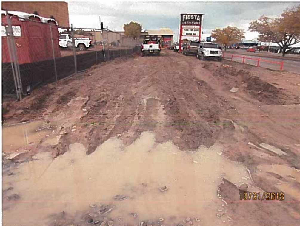
East exit with no track-out pad.
