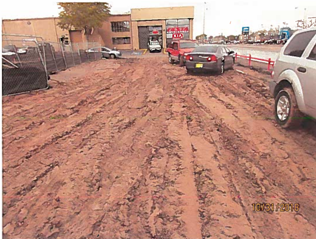
Muddy parking area. Mud being tracked off-site.
