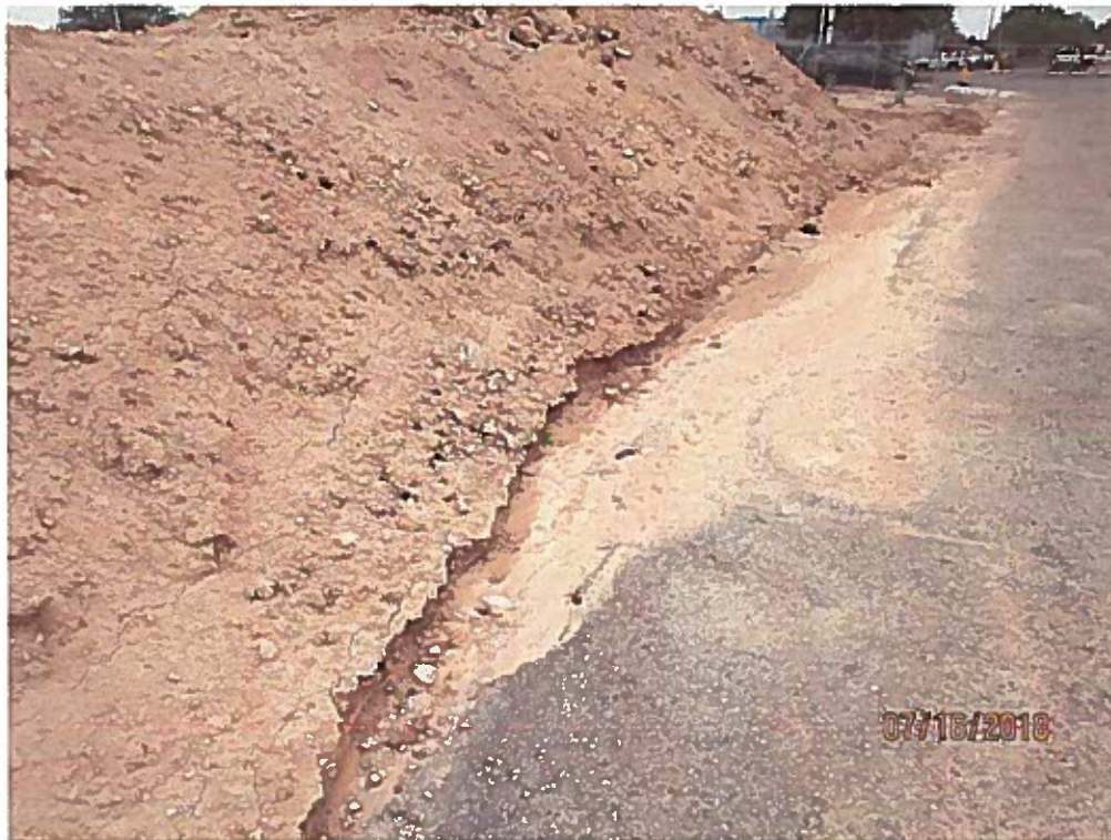
Close-up of stockpile erosion.
