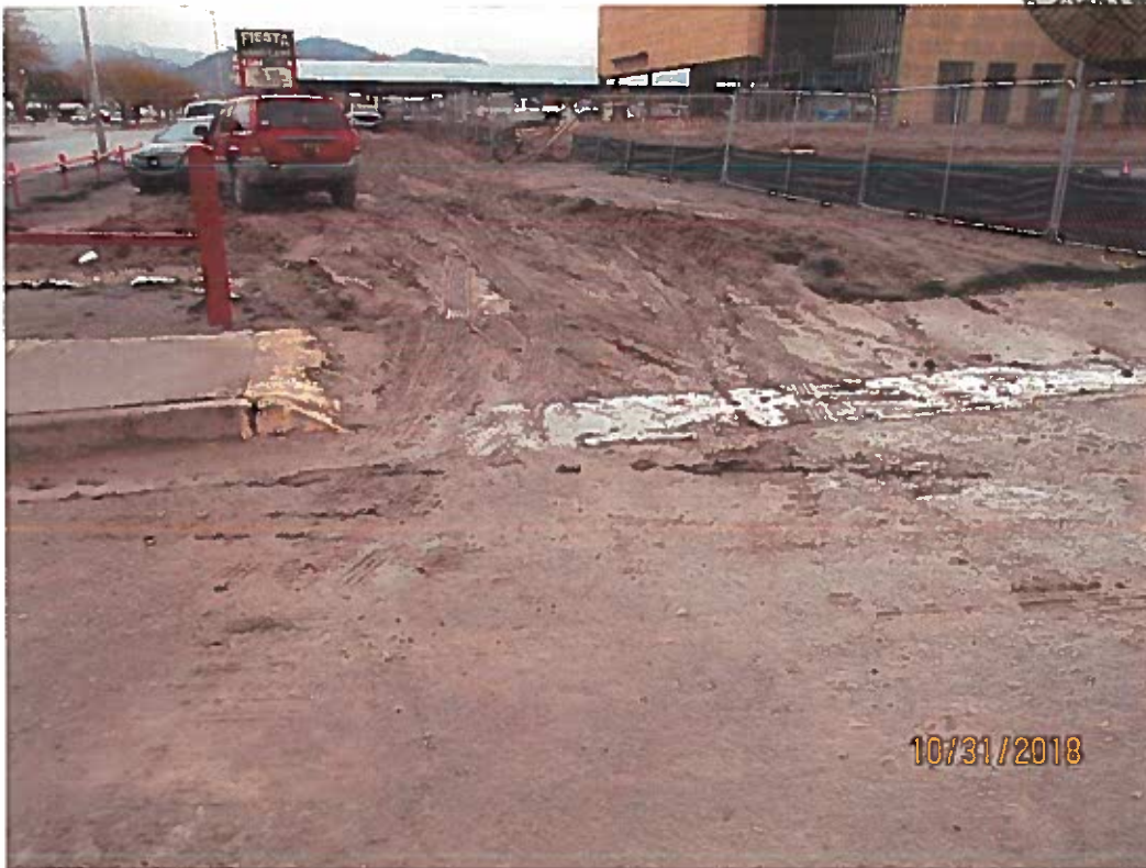
West exit with no track-out pad.
