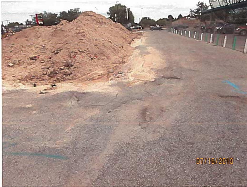
Area where off-site flows entered the site and eroded the stockpile.
