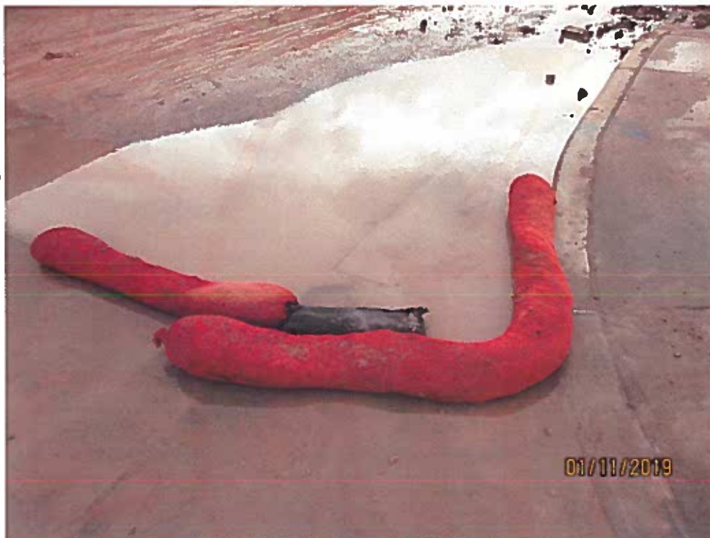
The City deployed BMPs to help mitigate the amount of sediment entering Lomas Blvd.
