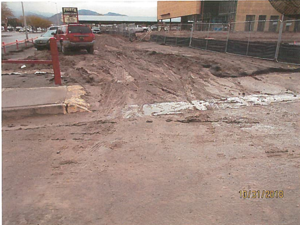
West exit with no track-out pad.
