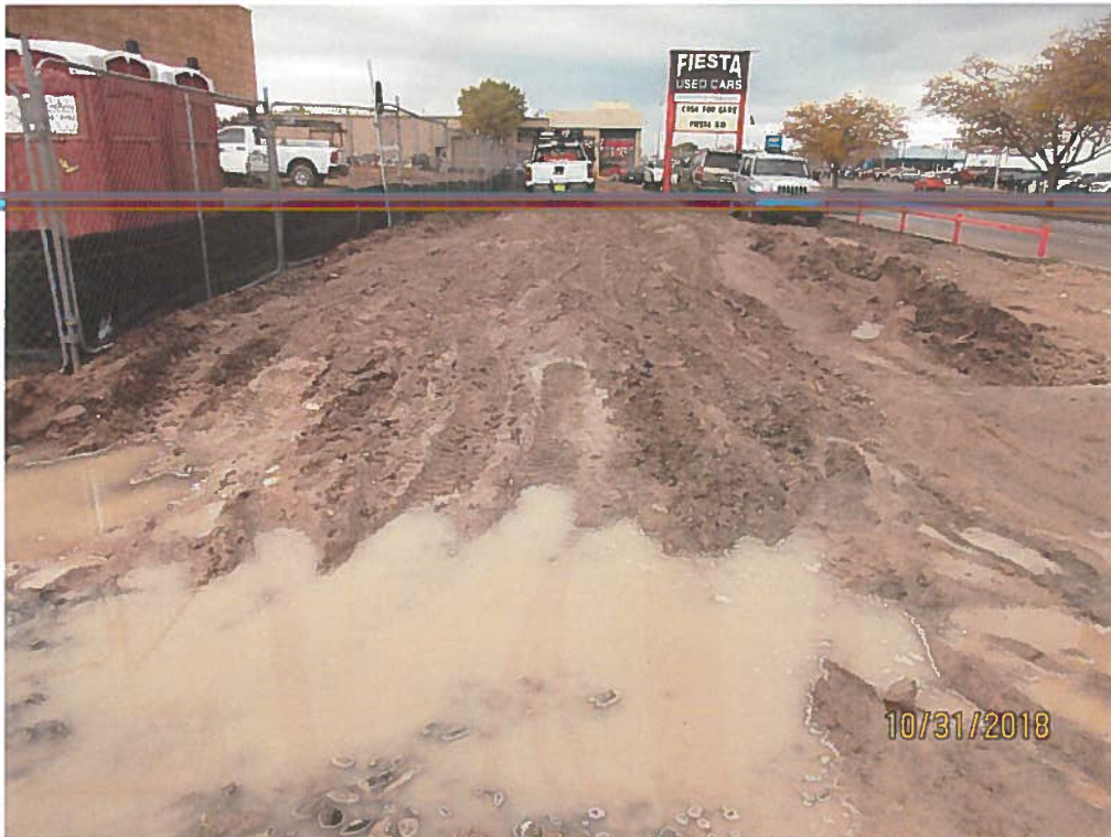
East exit with no track-out pad.
