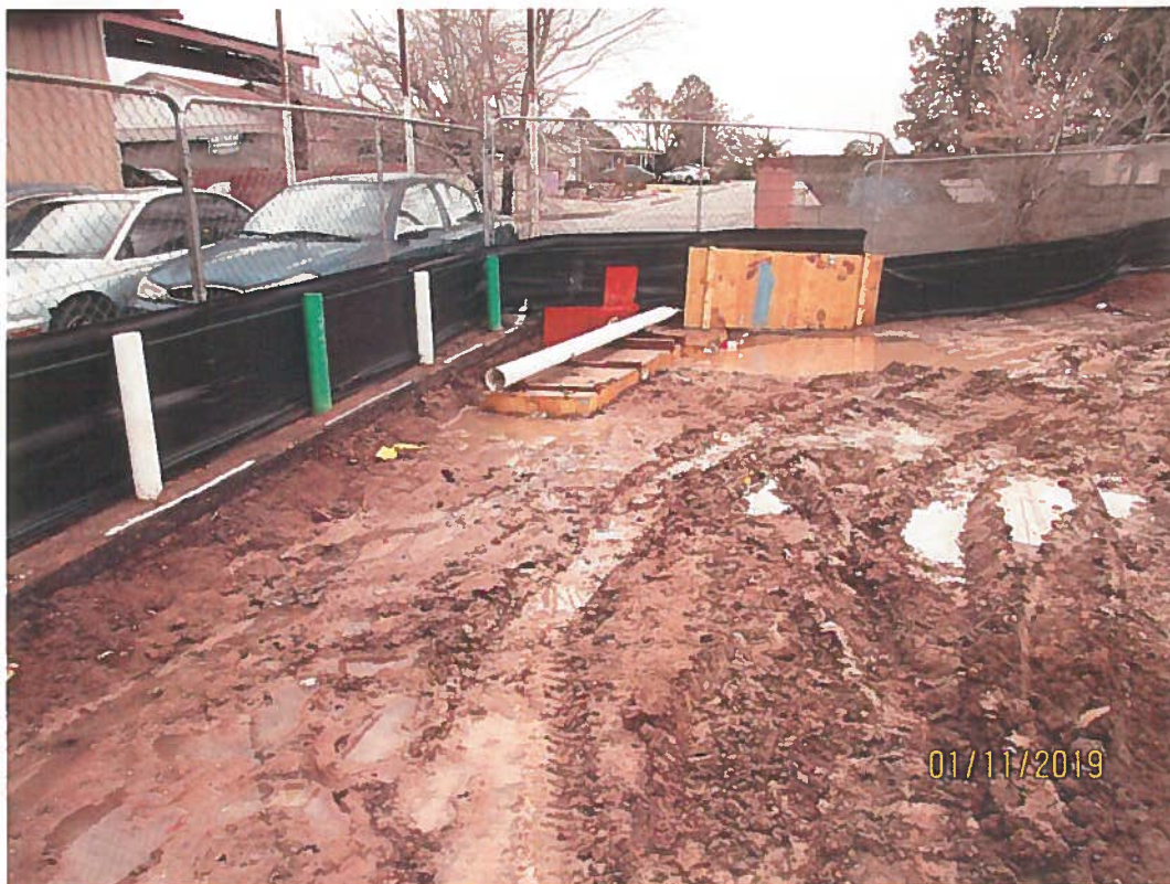
Pipe from offsite basin discharging into the site.
