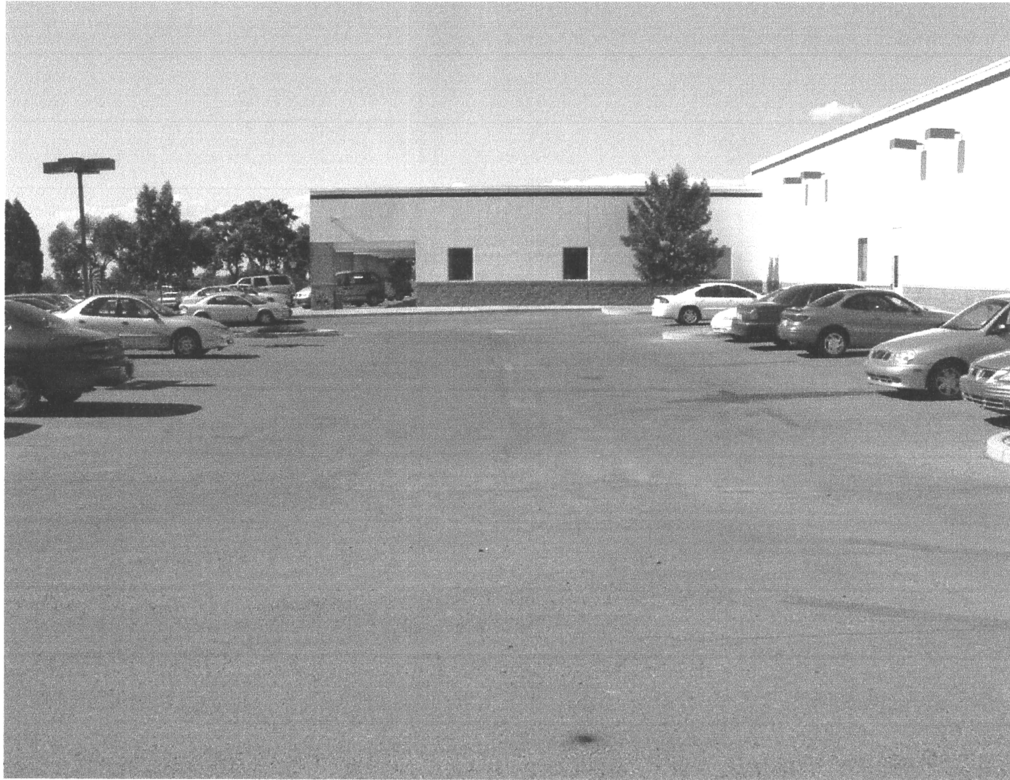
DriveTime Site – area of proposed building extension
