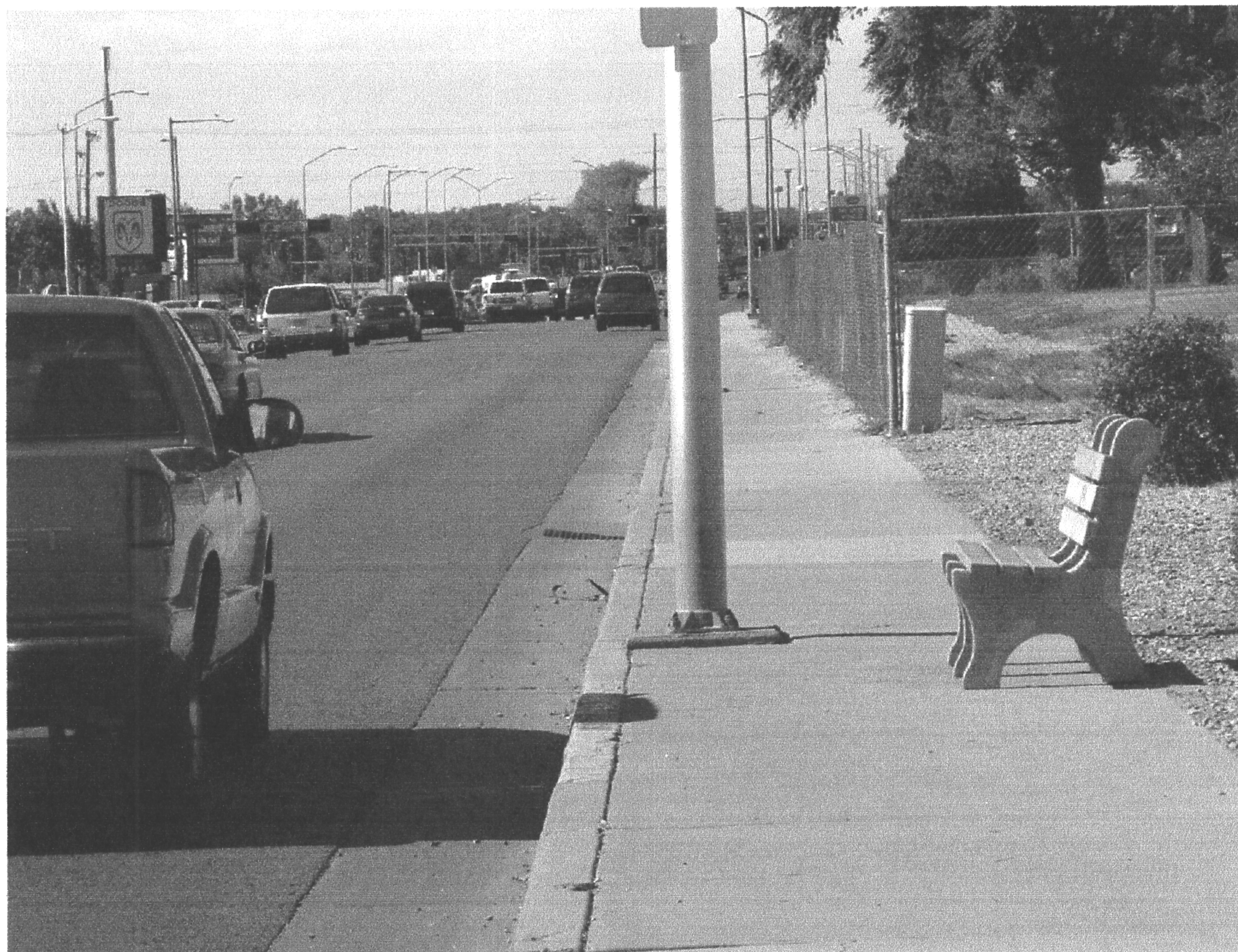
DriveTime Site – existing storm line drop inlet in Wyoming Blvd.
