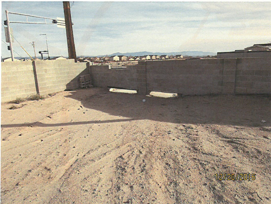
Holes in wall where sediment is leaving the property.
