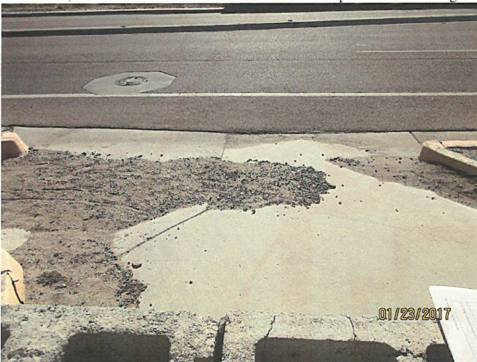
Sediment on ADA ramp/sidewalk.
