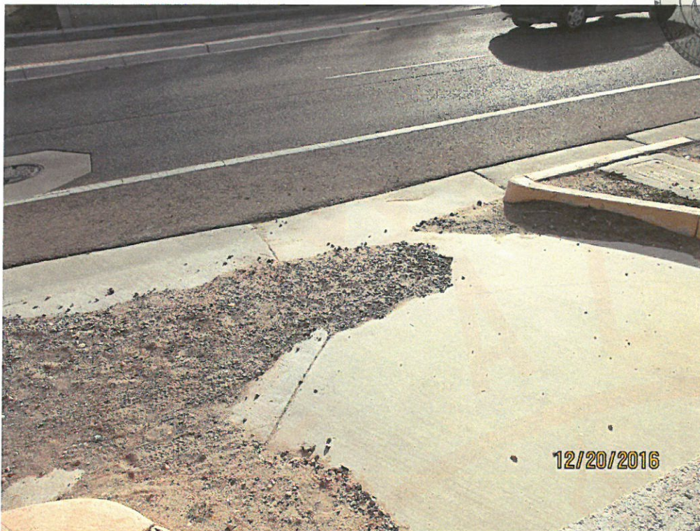
Sediment on sidewalk/ADA ramp on Sage Rd.
