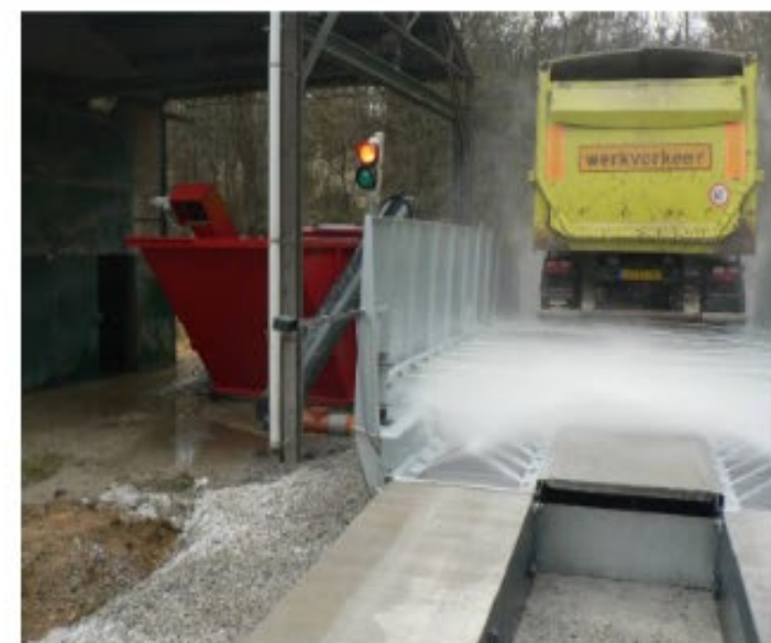
WHEEL WASH - PRESSURE WASHING DIRT OFF VEHICLE WHEELS CAN BE VERY EFFECTIVE. WHEEL WASH WASTEWATER IS PROCESS WATER, NOT STORMWATER. IT MUST BE DISCHARGED TO A SEPARATE ON-SITE TREATMENT SYSTEM THAT PREVENTS ITS RELEASE FROM THE SITE.
