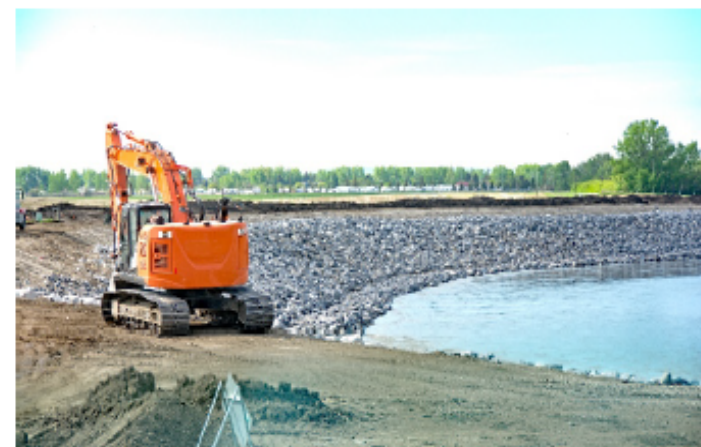
A riprap-lined bank surrounding a newly constructed detention pond.
