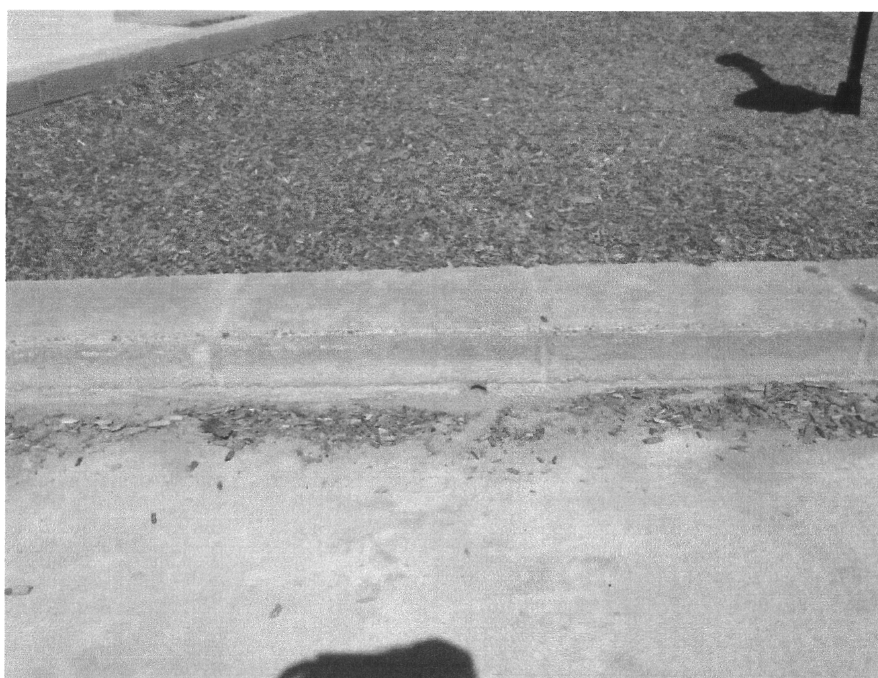
Figure 2. APS has drilled weep holes in the adjacent curb to drain the low point. Dirt and wood chips continually obstruct the weep holes.
