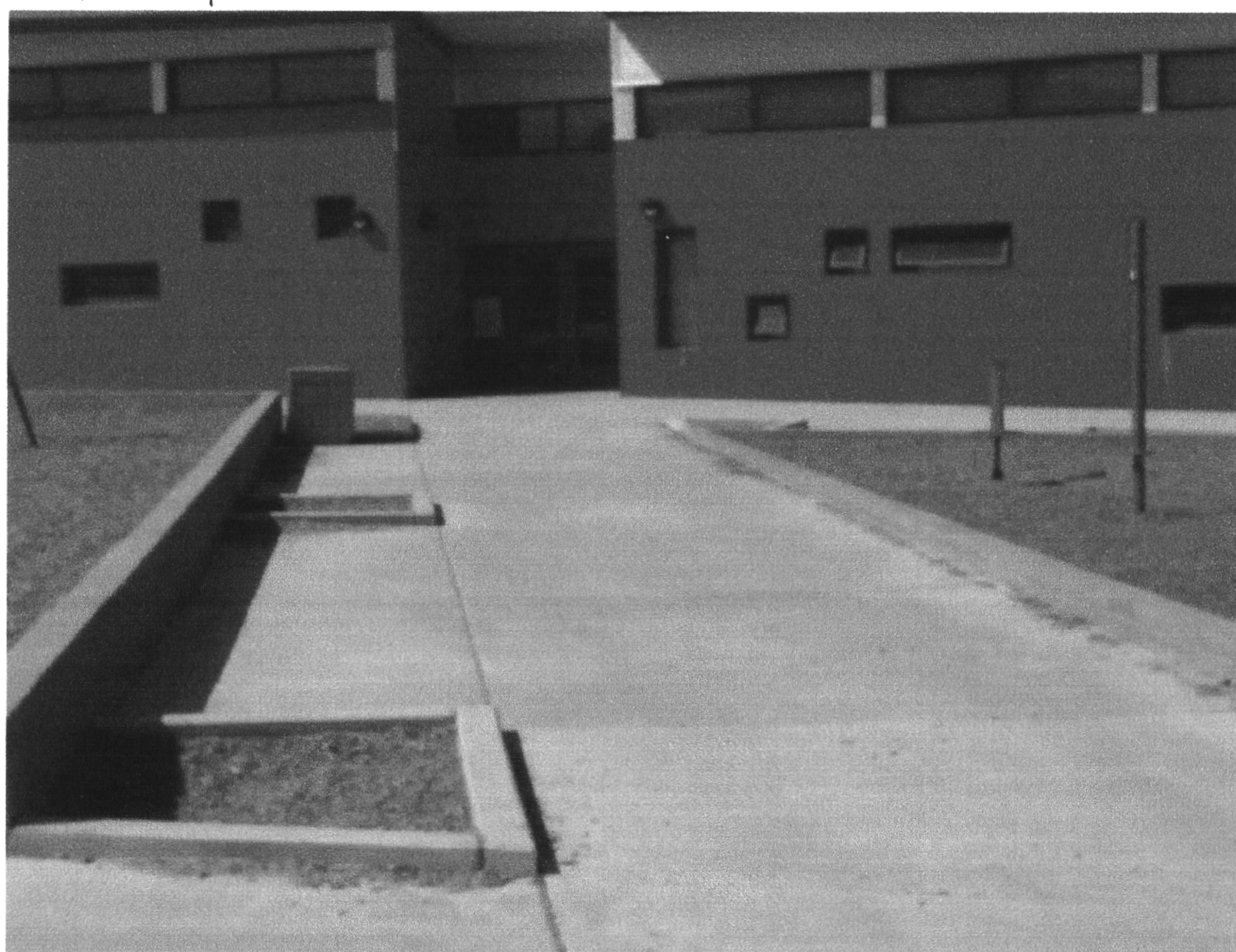
Figure 1. The sidewalk slopes down to a low point rather than high point as originally designed.
