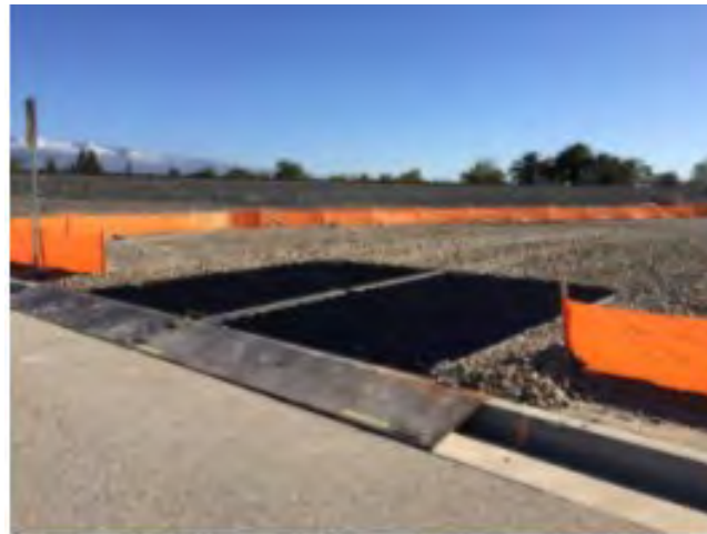
SEDIMENT TRACK OUT CONTROL
