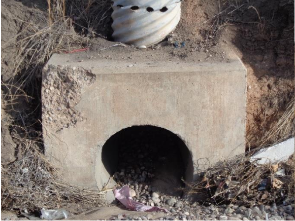
Figure 6 - Damaged Outfall
