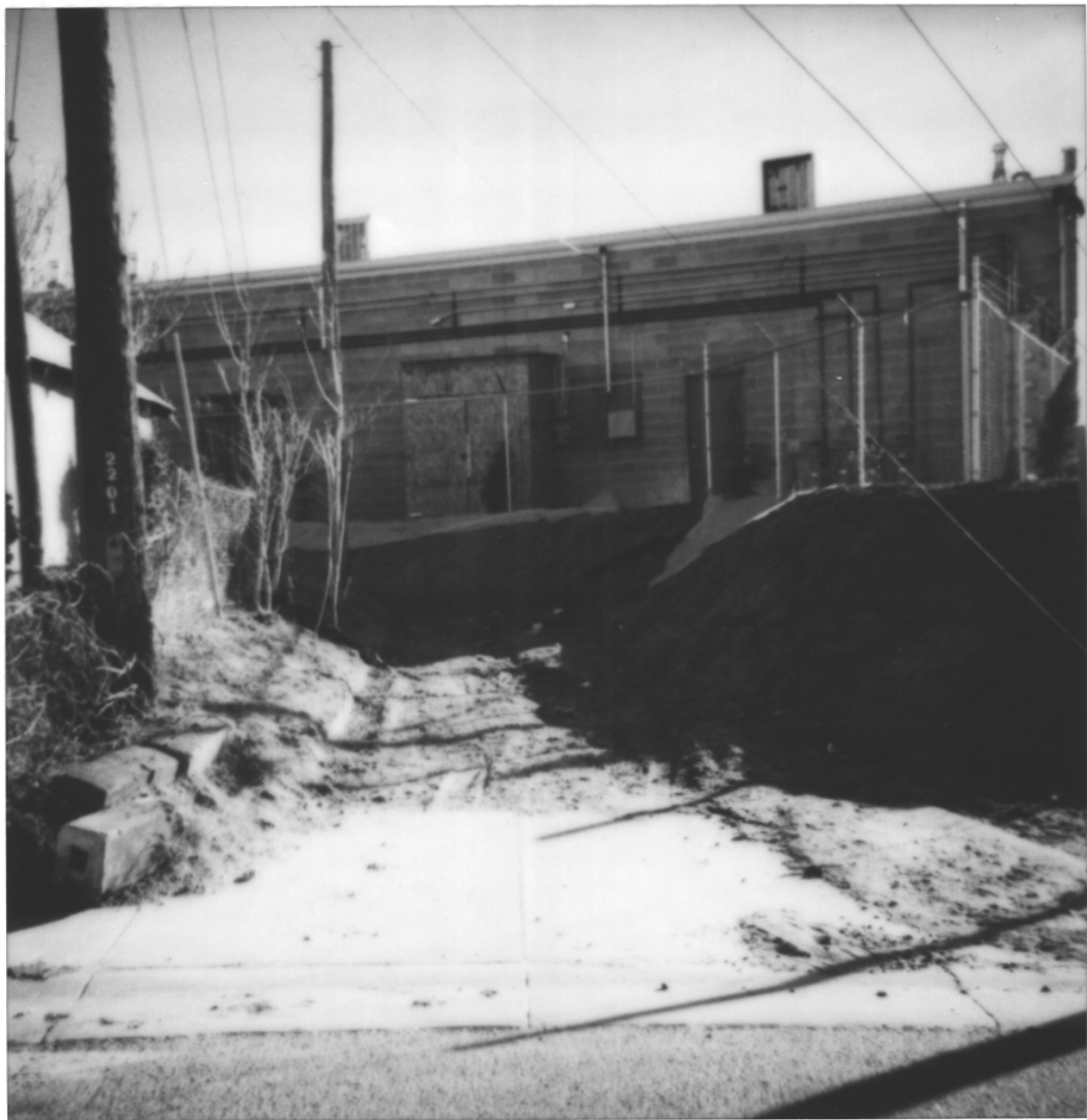
① Looking south on Ross Ave St. along 16' wide Alley.
