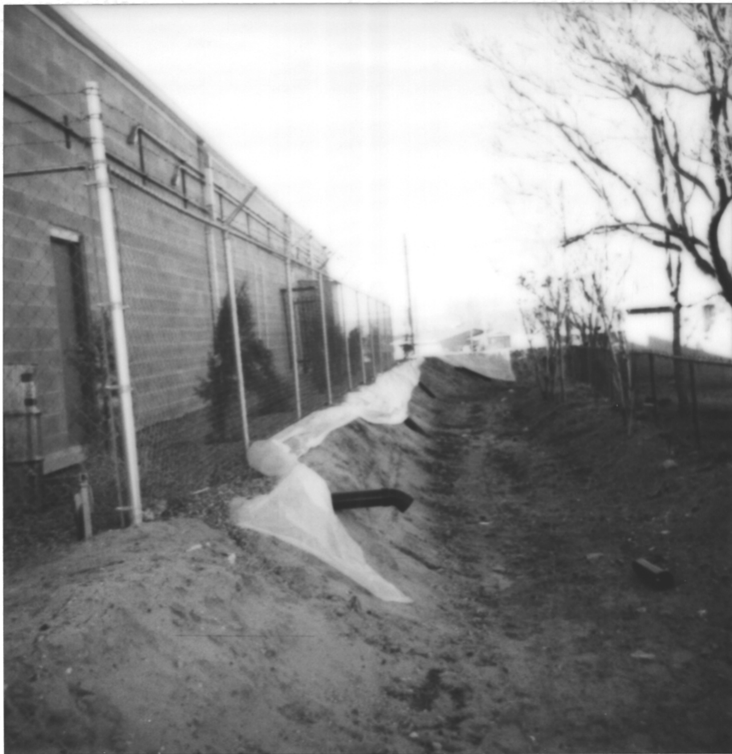
② Looking west on northeast corner of 16' Alley.
