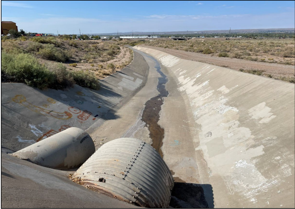
Photograph 1 Geneva's Arroyo channel facing downstream (westward) from the buried pipe outlet
