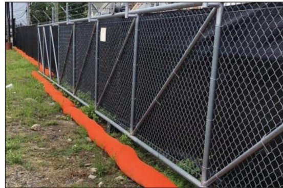
Filtrex SiltSoxx EXTREME used in rugged conditions.
