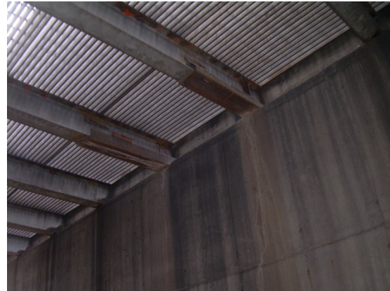
Steel plates were used to repair two girders at the west abutment
