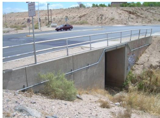
The superstructure has 22 steel "I" girders, type 12 WF 27. The girders are approximately 12 inches deep at 4-foot spacing. The girders support a 5-inch thick steel grate deck, which allows for through drainage. The beams are
