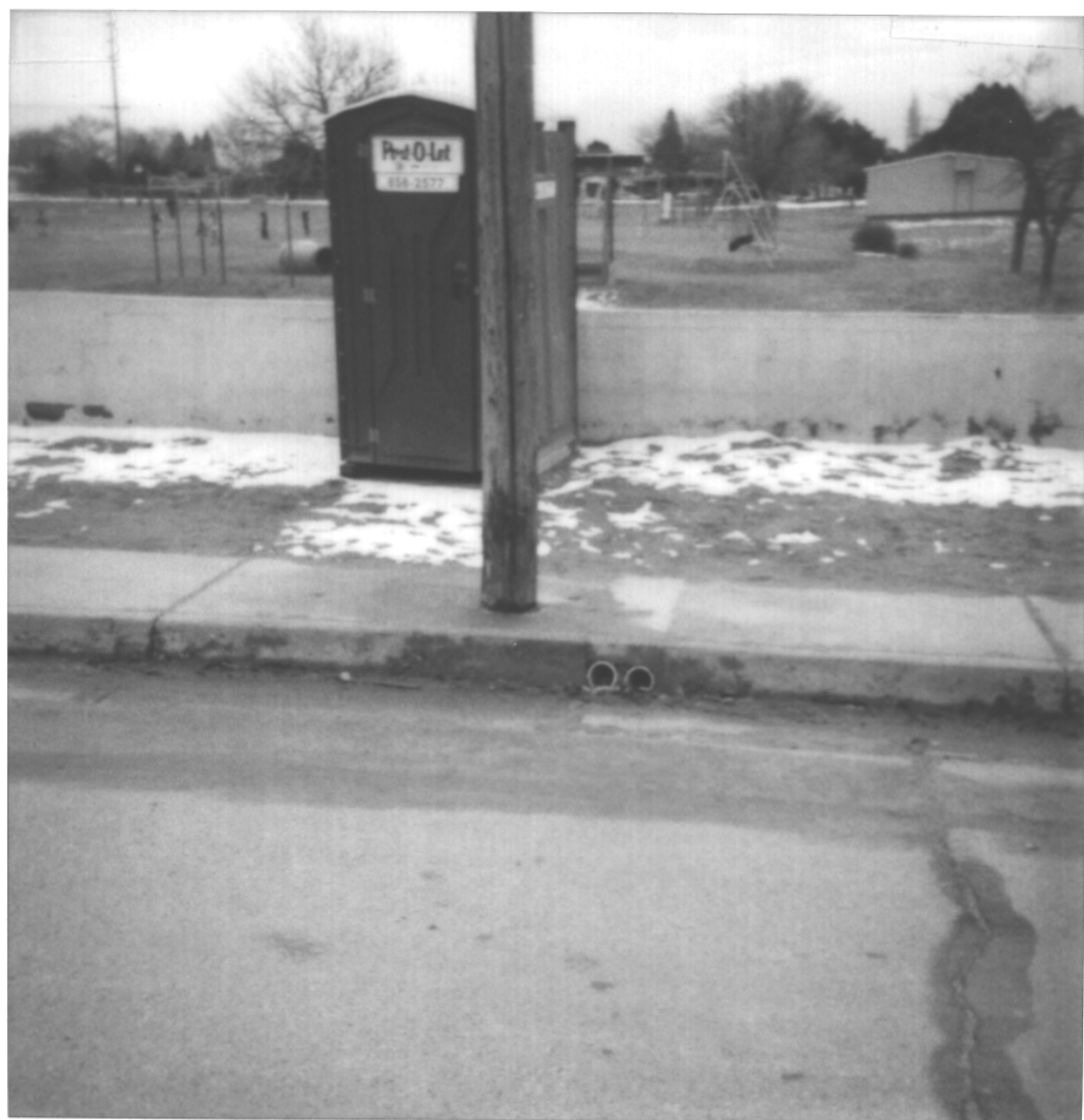
Outlet From 1-13-93 Catch Basin @ Tulane
