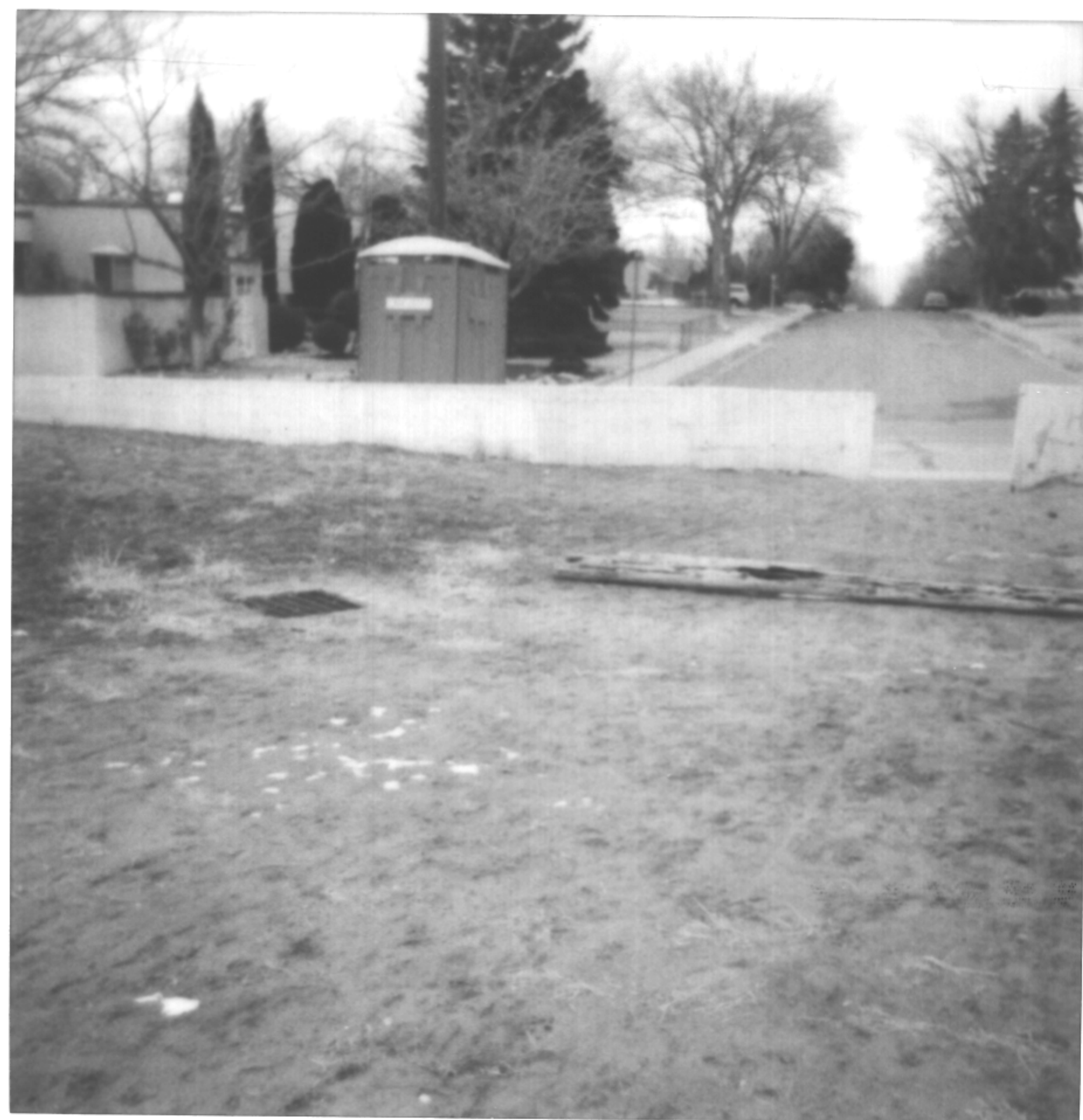
Catch Basin 1-13-93 @ Tulane
