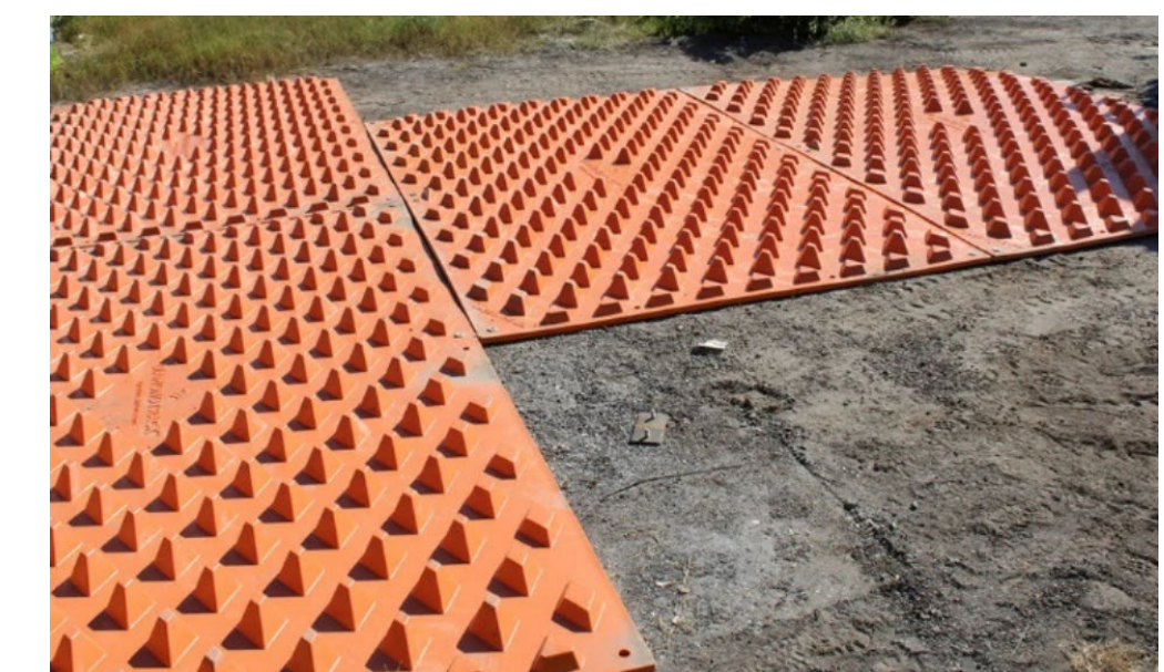
INSTALL FODS ACCORDING TO THE MANUFACTURER'S SPECIFICATIONS. FODS TRACKOUT CONTROL MATS CAN BE USED WITH A STABILIZED CE OR ALONE, AS LONG AS THEY CAN ACCOMMODATE THE TURNING MOVEMENTS OF THE LARGEST VEHICLES EXITING THE SITE.
