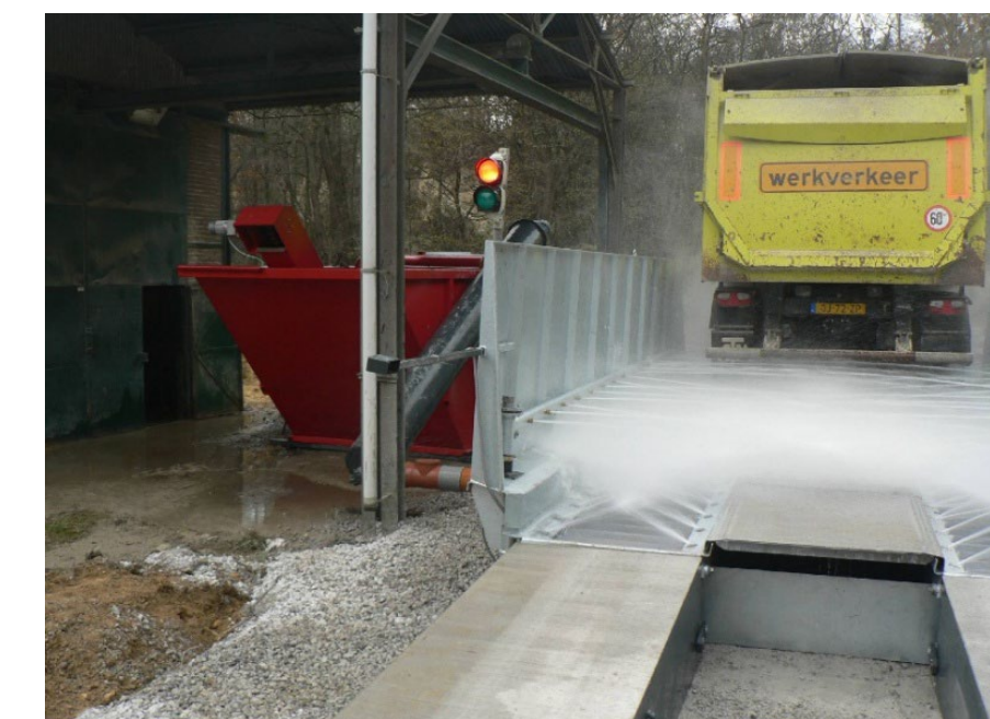
WHEEL WASH - PRESSURE WASHING DIRT OFF VEHICLE WHEELS CAN BE VERY EFFECTIVE. WHEEL WASH WASTEWATER IS PROCESS WATER, NOT STORMWATER. IT MUST BE DISCHARGED TO A SEPARATE ON-SITE TREATMENT SYSTEM THAT PREVENTS ITS RELEASE FROM THE SITE.
