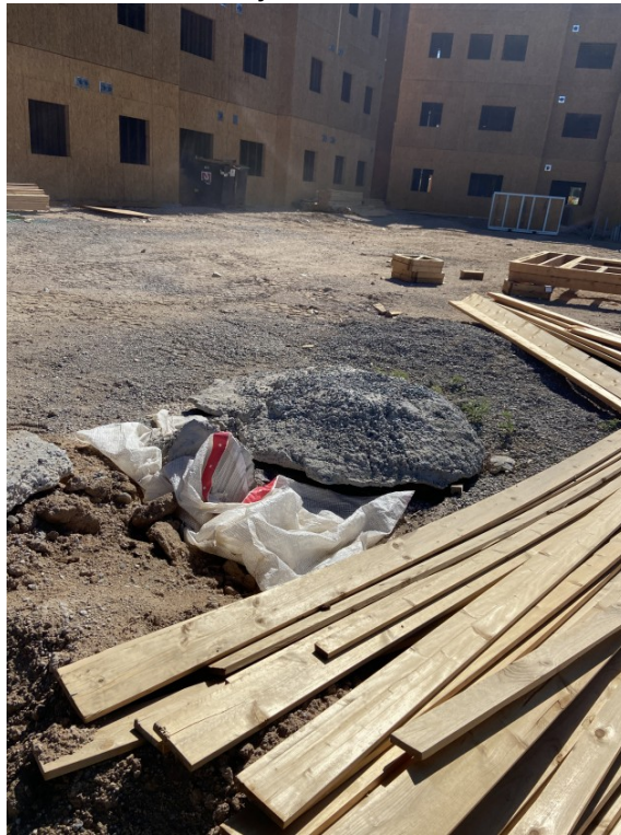
Site Walk Deficiency Photos - Concrete washout
