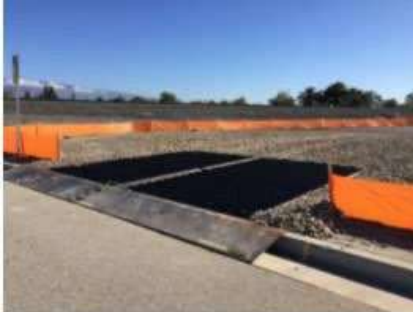
SEDIMENT TRACK OUT CONTROL
