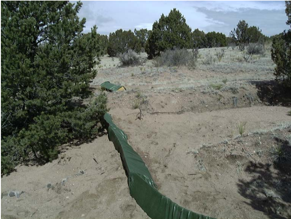
Triangular sediment filter dike
