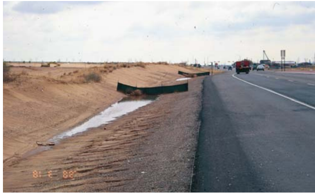
Check dams at roadside ditch
