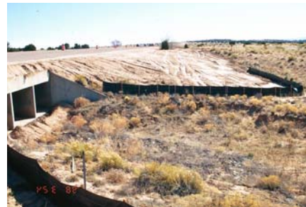
Silt fence at outlet of box
