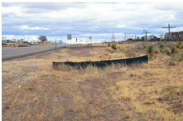
Check dam at roadside ditch
