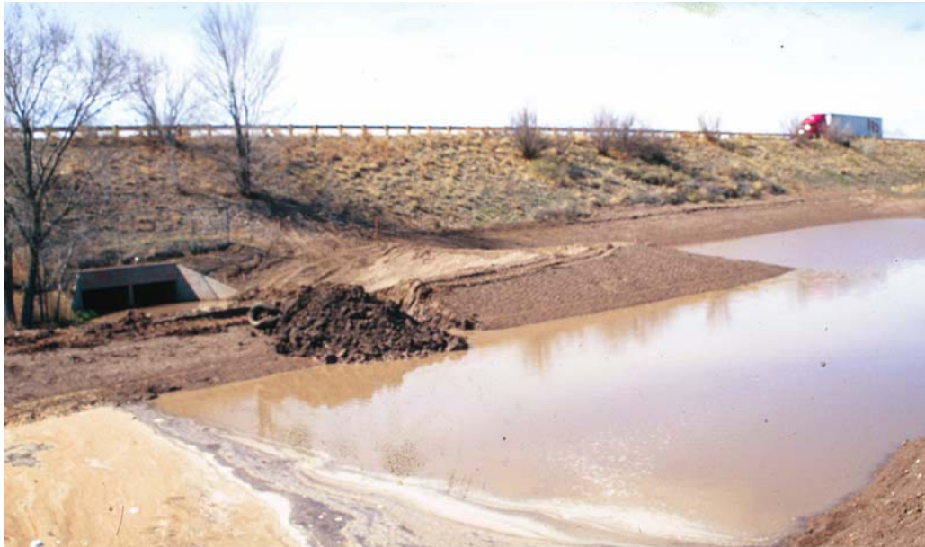
Sediment pond at inlet of box
