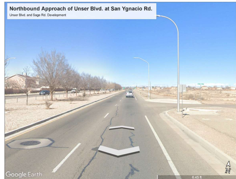
Figure 36: Northbound Approach Streetview of Unser Blvd. at San Ygnacio Rd.
