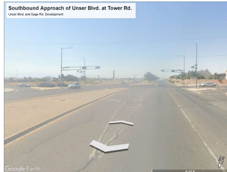
Figure 22: Southbound Approach Streetview of Unser Blvd. at Tower Rd.
