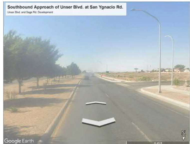
Figure 37: Southbound Approach Streetview of Unser Blvd. at San Ygnacio Rd.
