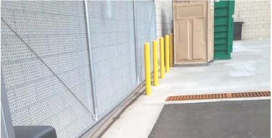
12. The large paved area to the east of the trash area is covered by a roof which is not shown on the plans. It appears to drain the same direction as the concrete area shown on the plans.
