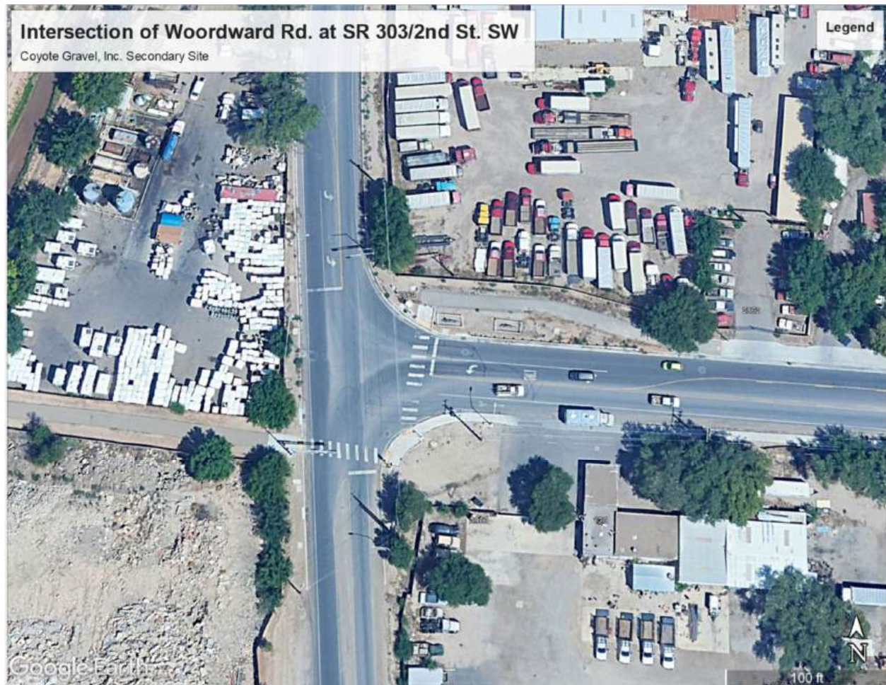
Figure 12: Signalized Intersection of Woodward Rd. SW at SE 303/2nd St. SW
