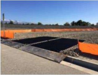
SEDIMENT TRACK OUT CONTROL
