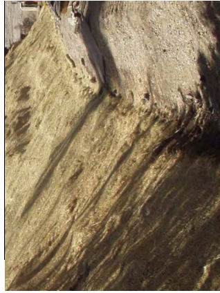
BERMS AND SWALES
