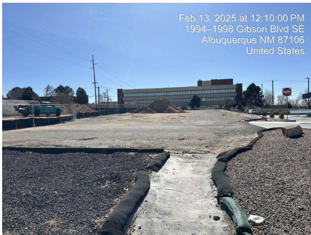
2Inlet with no protection from the exposed stockpile
